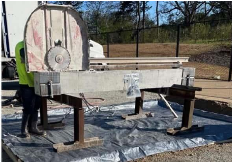
Figure 4-16 Track saw mounted on beam
