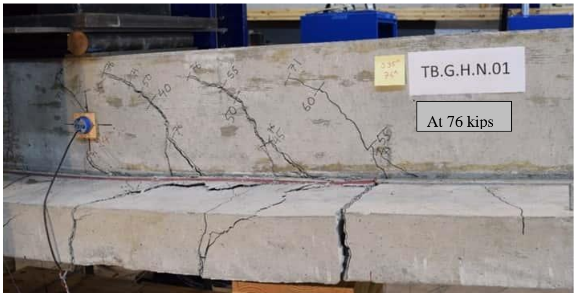
Figure 7-6 Crack formation at the hook and delamination for Specimen TB.G.H.N.01
