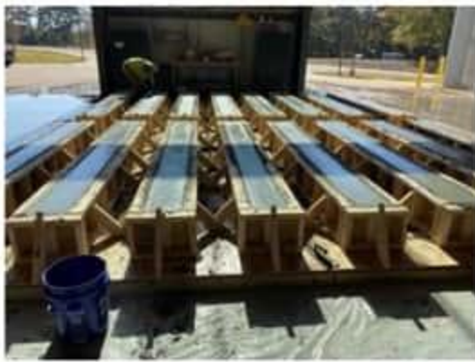
Figure 4-8 Beam after placement (Left) and moist curing (Right)
