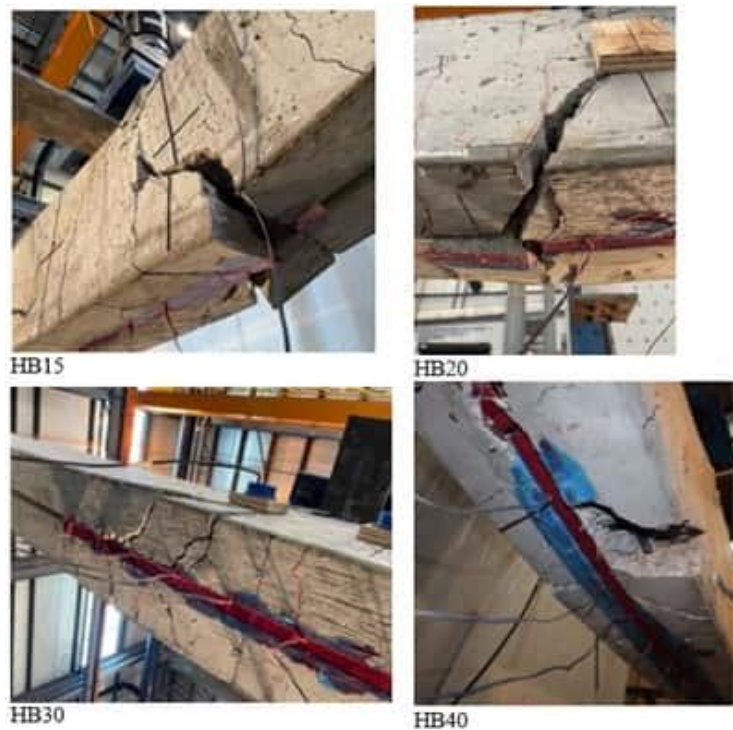
Figure 5-7 Post-test specimen pictures of anchorage failure (HB 15 and HB20) or concrete-epoxy interface failure (HB30 and HB40)
