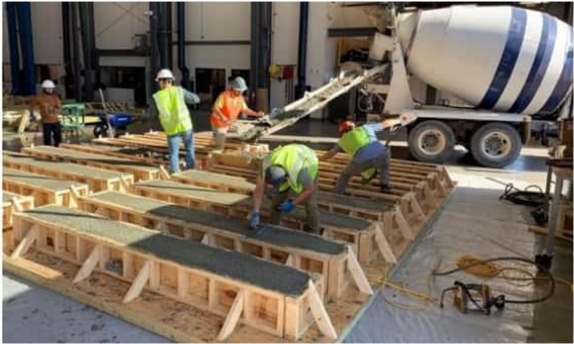
Figure 4-6 Concrete casting, vibrating and finishing
