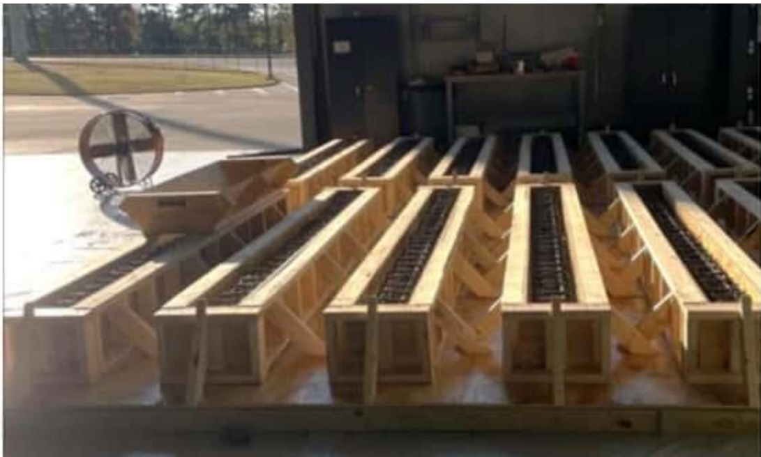
Figure 4-5 Concrete forms and sliding funnel
