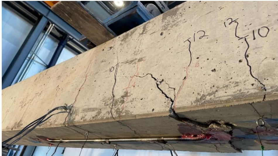
Figure 5-24 Inclined cracks formation near hook ends of HU30
