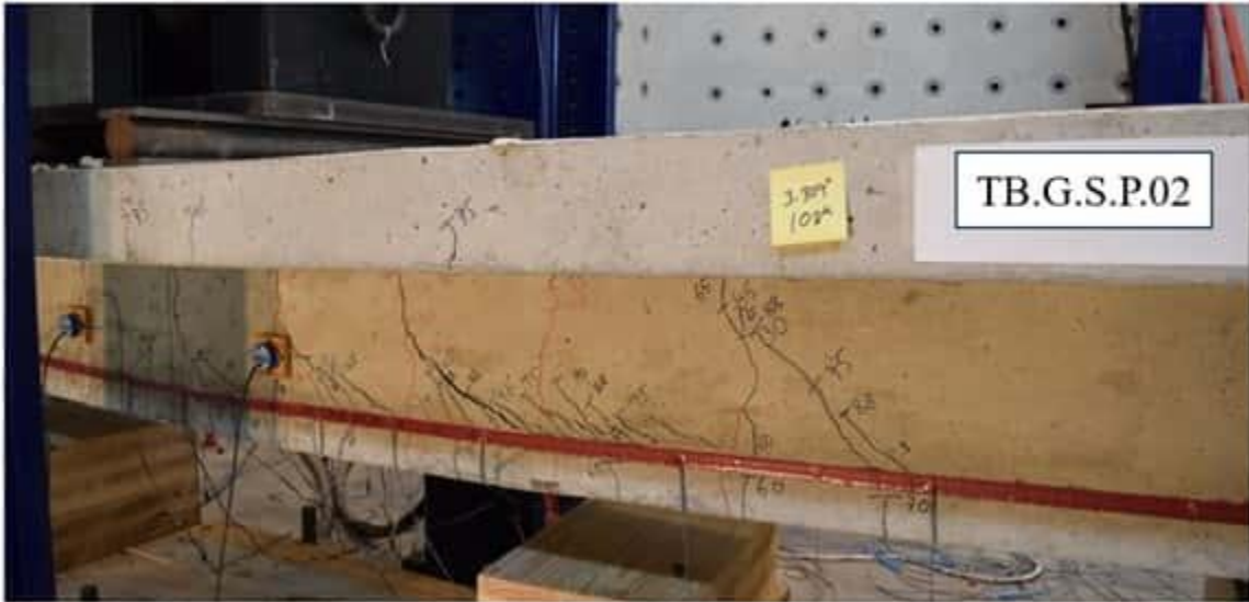
Figure 7-11 Concrete-epoxy interface failure for Specimen TB.G.S.P.02 at 108 kips load
