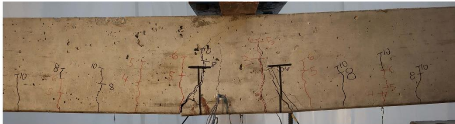
a) Inclined cracks at hook ends (12.7 kips)
