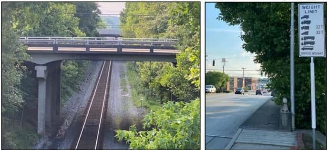
Figure 1-1 Picture of the Cullman Bridge and the Posted Weight Limit Sign
