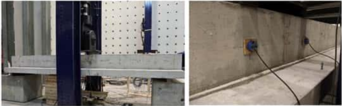
(a) Specimen for cracking
