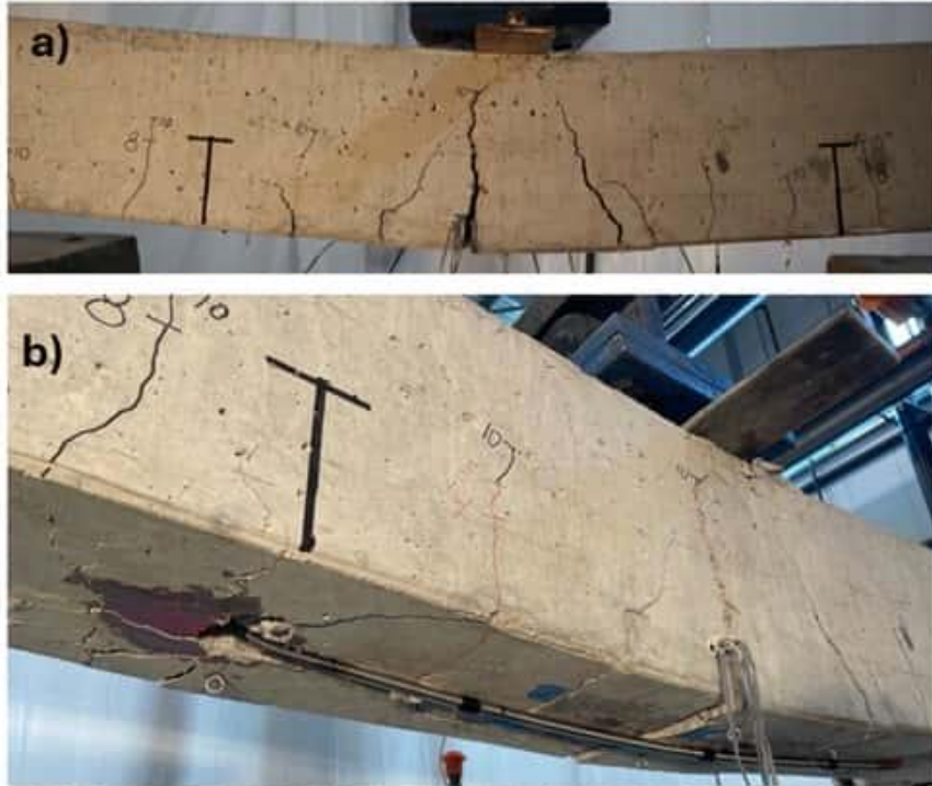
Figure 5-25 a) Widened and inclined cracks in the central region and b) widened cracks near hook ends of HU40
