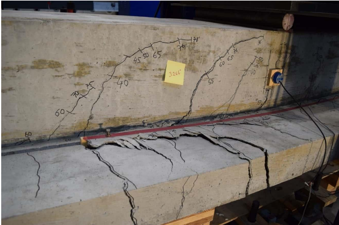
Figure 7-13 Wide crack formation at the end of TiAB and concrete-epoxy interface delamination for Specimen TB.G.S.N.01
