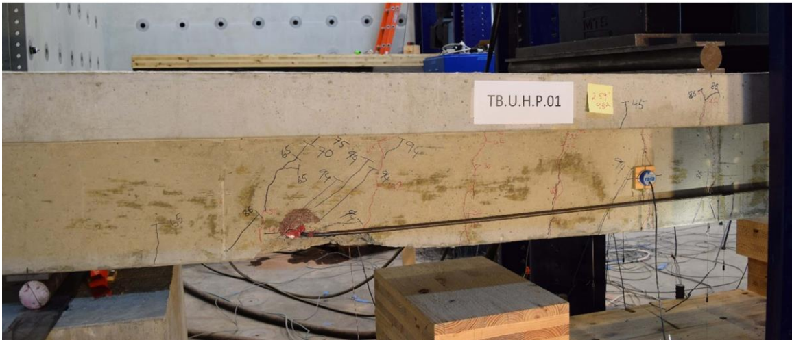
Figure 7-16 Anchorage failure of Specimen TB.U.H.P.01
