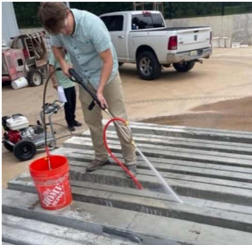
Figure 4-18 Low-pressure water blasting with abrasives
