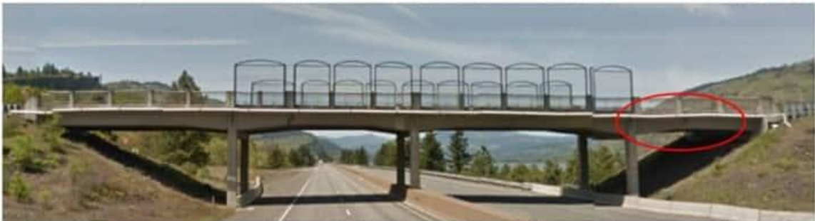
Figure 2-11 Mosier Bridge with Critical Section circled (Higgins, Amneus, Barker, 2015)
