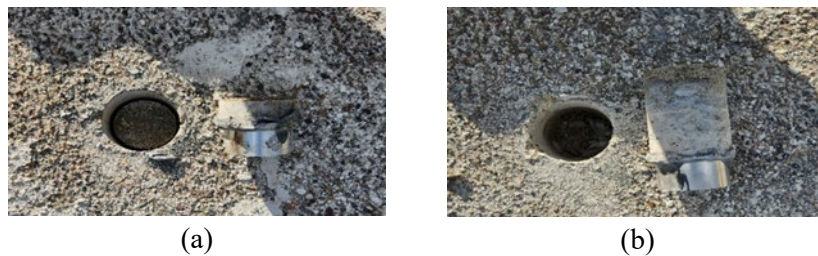
Figure 7.4 Failure modes recorded during bond strength tests a) bond failure and b) failure in substrate
