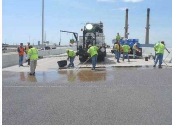
Figure 2.1 Overlaying concrete bridge deck with polymer concrete [23]
