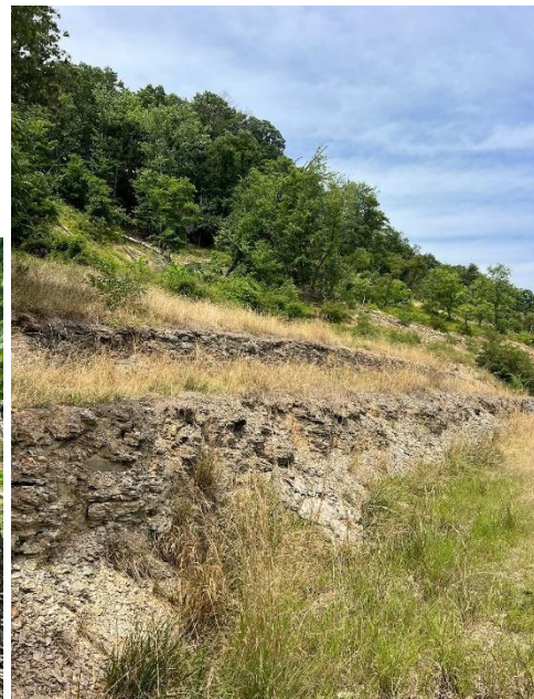
Figure 3.15: Starting point of landslide at the top (left) and benches built during the mitigation.
