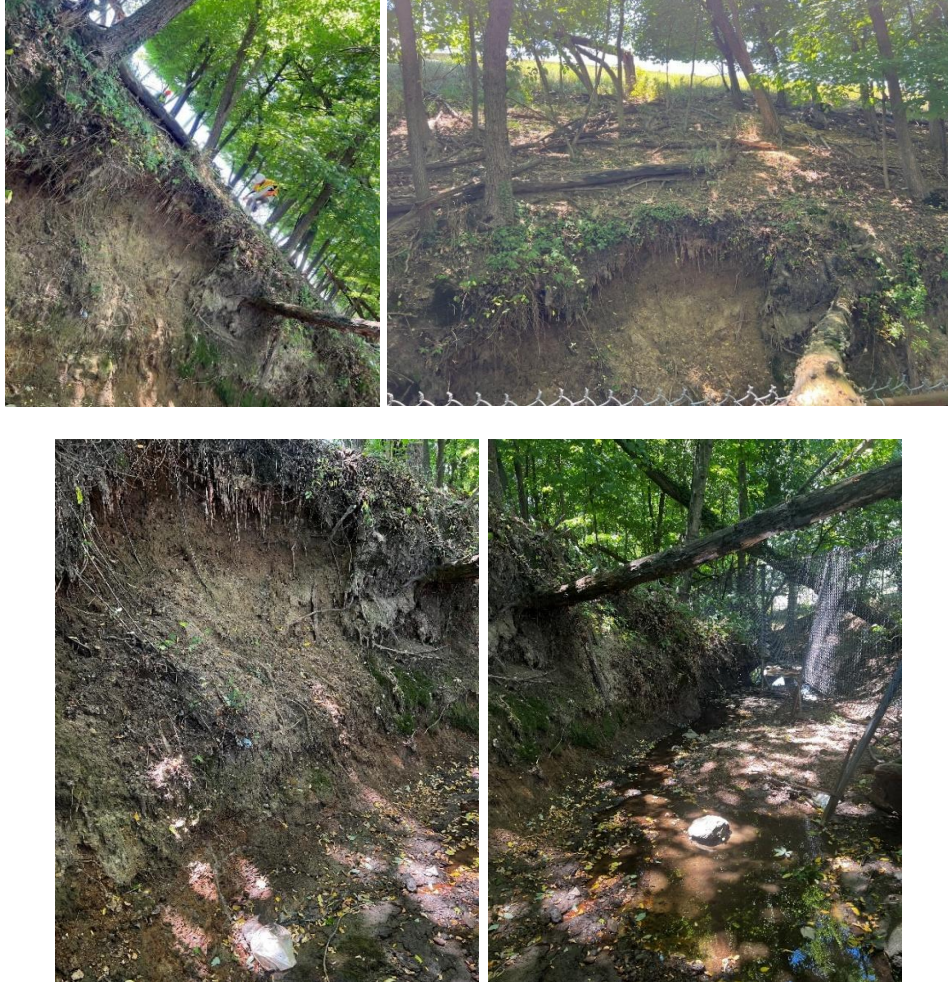
Figure 3.7: Site 2 landslide looks active and needs immediate attention.
