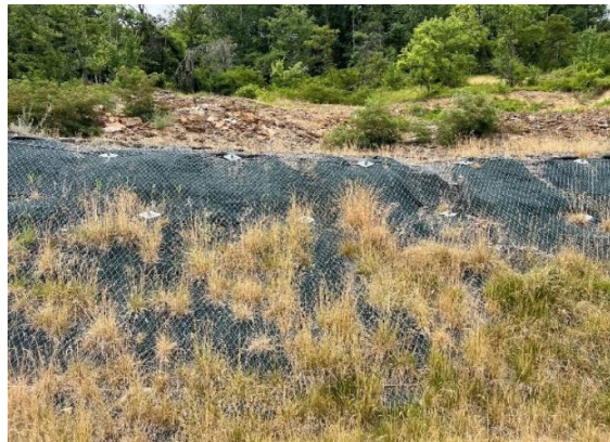
Figure 3.14. Soil nailing to mitigate landslide at site 13.
