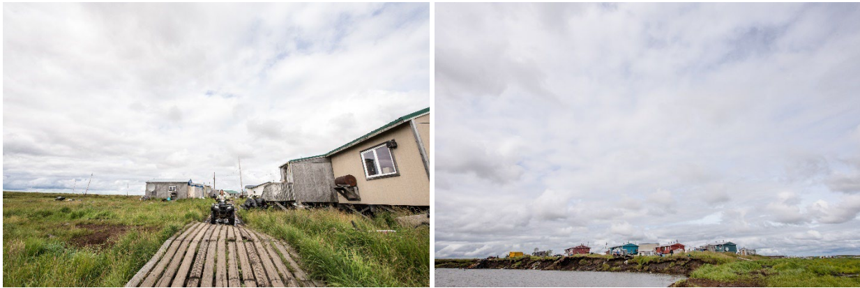
Figure 20. Boardwalks serve as roads in Newtok (left) as the ground is unstable or prone to erosion (right).
