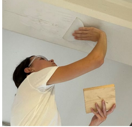
(c) Skim coat the surface of the substrate with epoxy.
