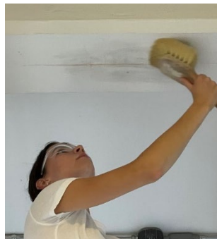
(b) Brush debris from the surface of the substrate.
