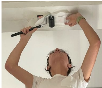
(b) Using a rubber roller, roll over the sensor to ensure adhesion.
