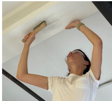
(a) Wire brush the surface of the substrate.
