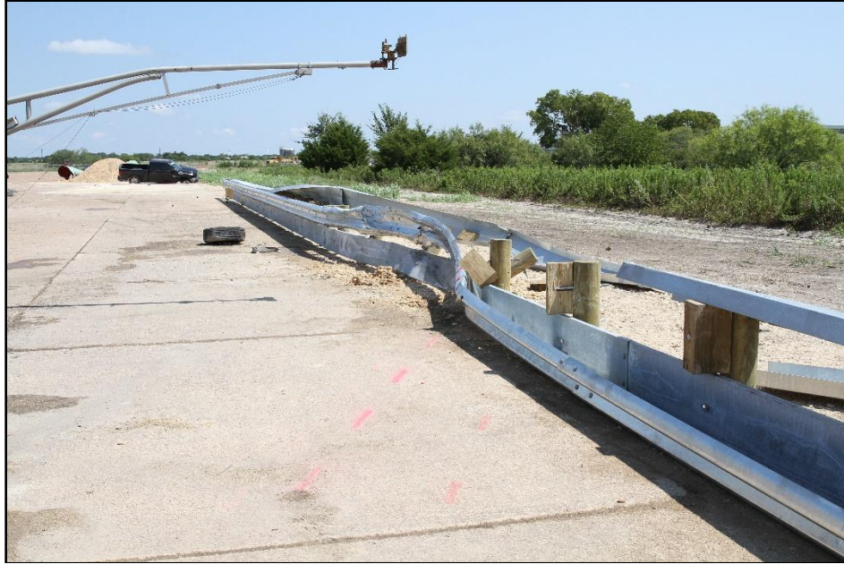
Figure 10.5. Enhanced Motorcycle Guard Fence System at Impact Location on the Traffic Side after Test 469940-03-2.
