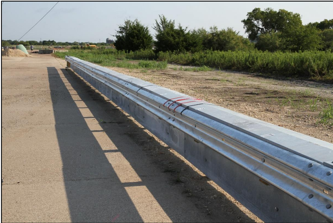
Figure 6.2. Enhanced Motorcycle Guard Fence System prior to Testing for 469940-03-1, 469940-03-2, 469940-03-3, and 469940-03-4A.
