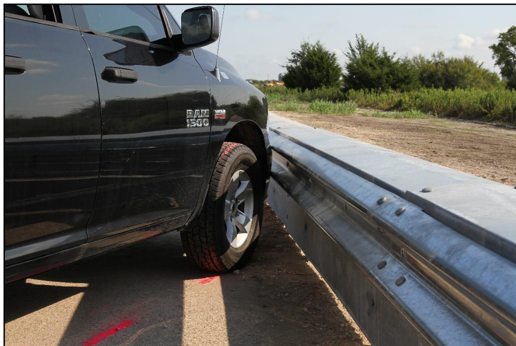
Figure 10.2. Enhanced Motorcycle Guard Fence System/Test Vehicle Impact Location for Test 469940-03-2.
