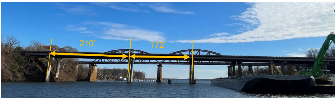
Figure 26. The bridge and the monitored spans with their length from the harbor deck's view
