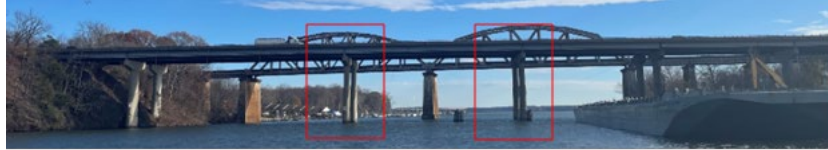
Figure 8. Occoquan bridge and target piers shown by red rectangles.
