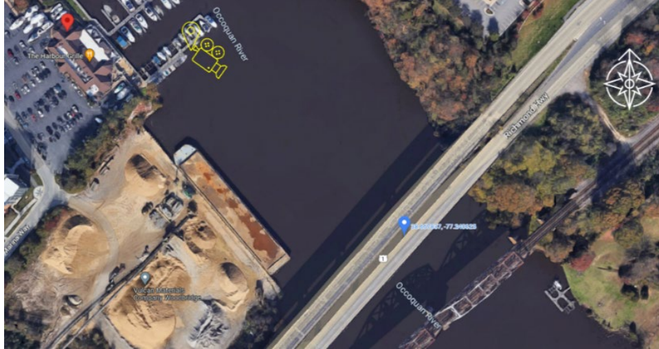
Figure 25. Aerial Google view of the bridge and the location of the deployments of the DMS
