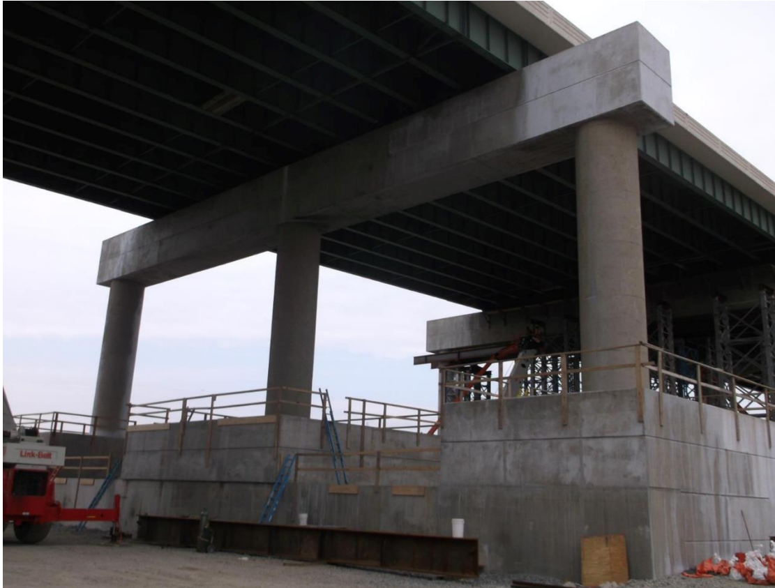
Figure 3-9 Permanent Completed Repairs (Benton, 2014)
