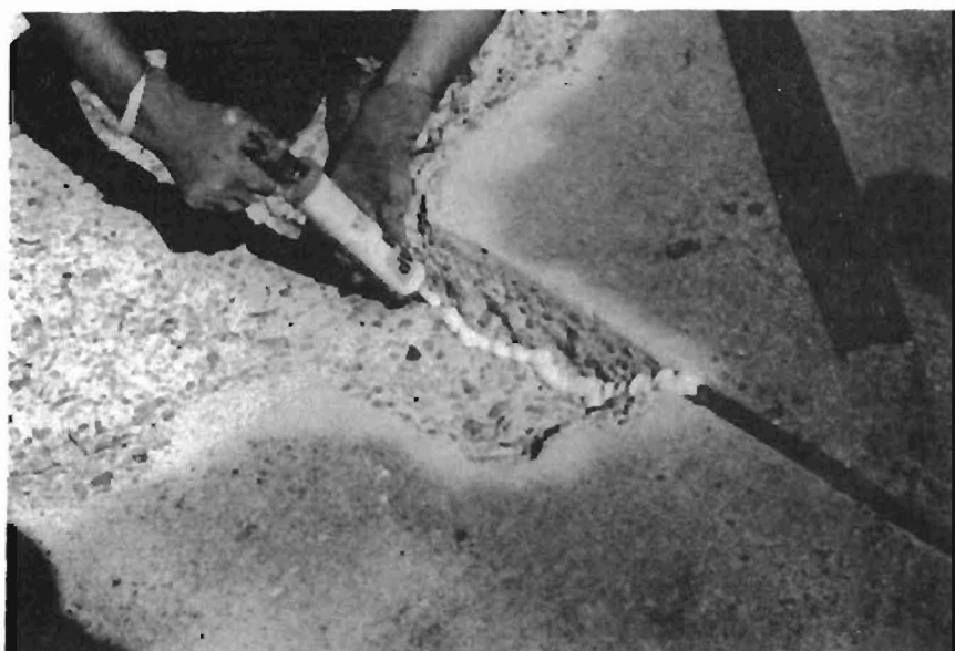
Fig. 4.3 Caulking Joints to Prevent Monomer Leakage.
