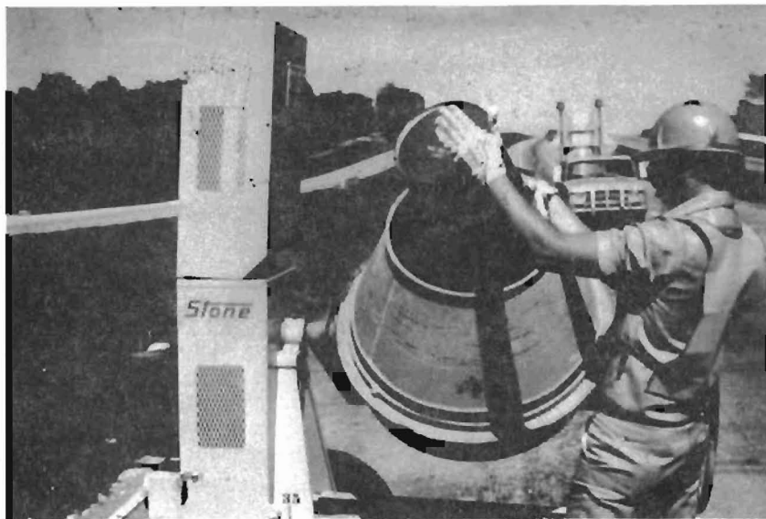
Fig. 4.7 Adding Liquid Component to Mixer.
