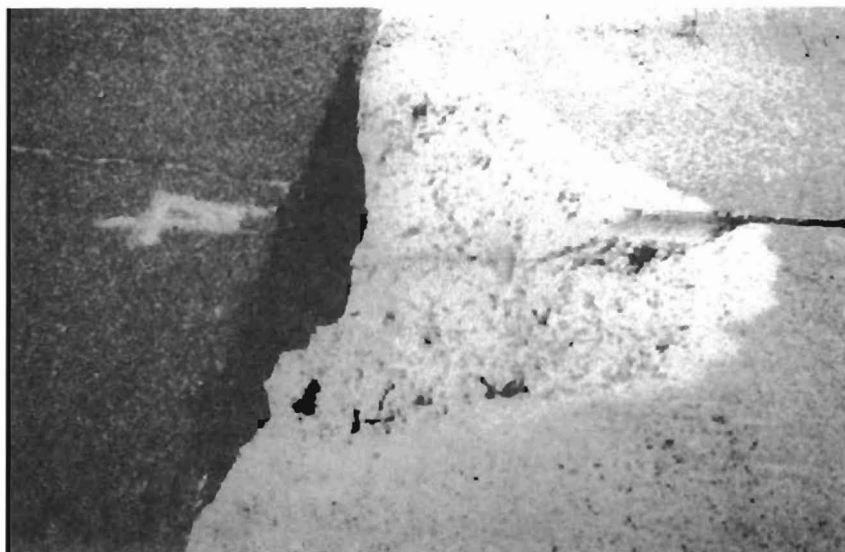
Fig. 4.2 Repair Area After Sandblasting.
