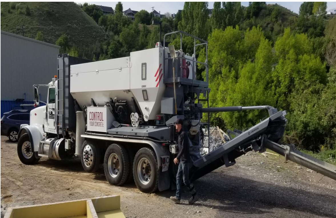
Figure 4.6: Volumetric concrete mixing truck
