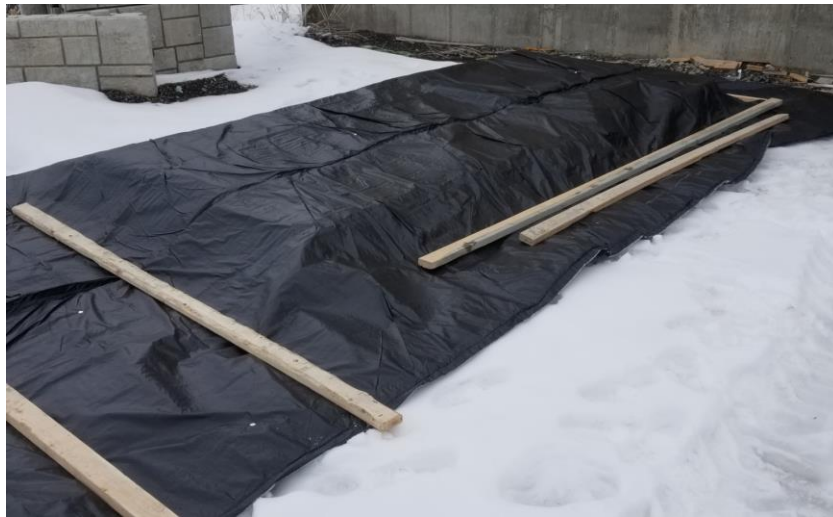
Figure 4.11: Curing of specimens under concrete blanket
