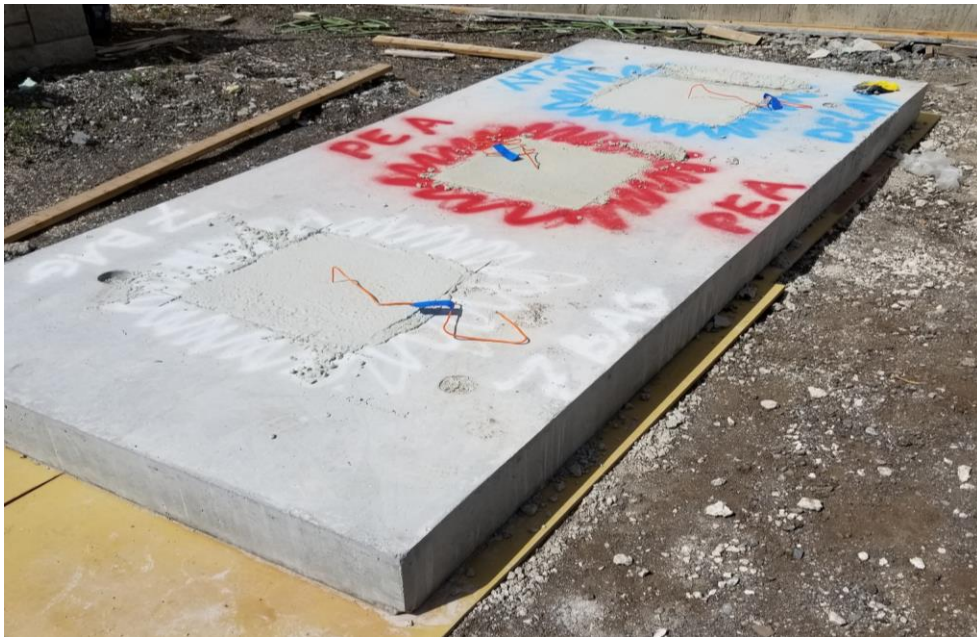
Figure 4.14: Color labeling on 6'x14'x9" small pavement repair slab
