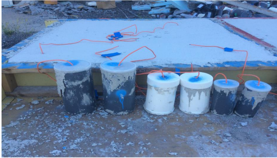
Figure 4.12: TMM sensors embedded in reference cylinders
