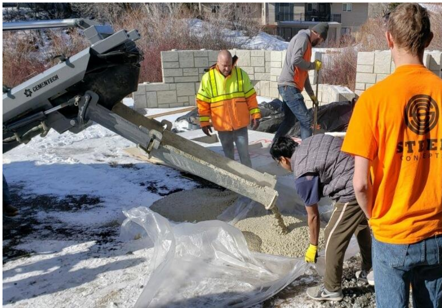
Figure 4.9: Concrete used to fill cylinders
