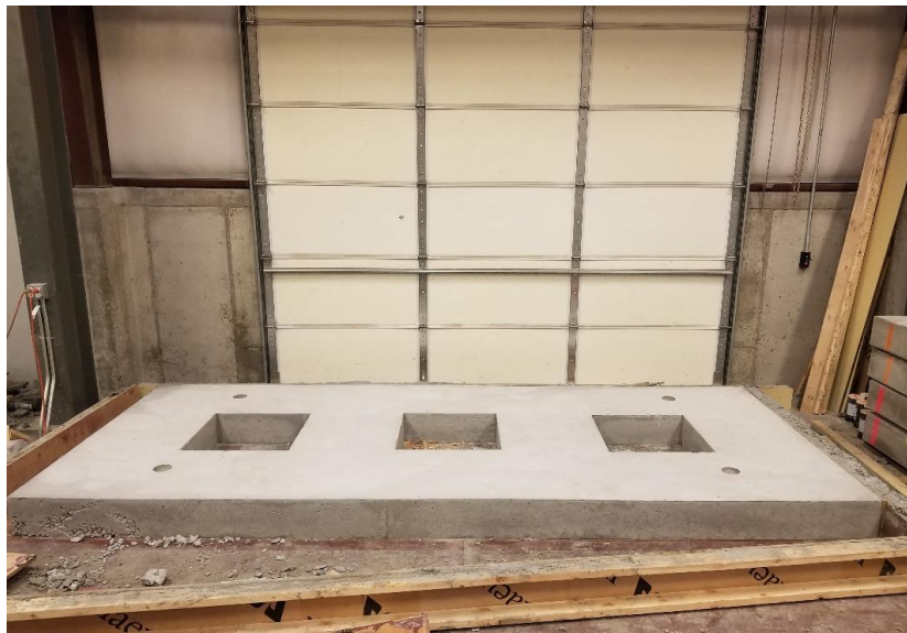
Figure 4.5: Concrete pavement repair slab normalized to controlled ambient air conditions
