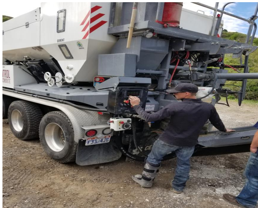
Figure 4.8: Adjusting the mix to increase slump
