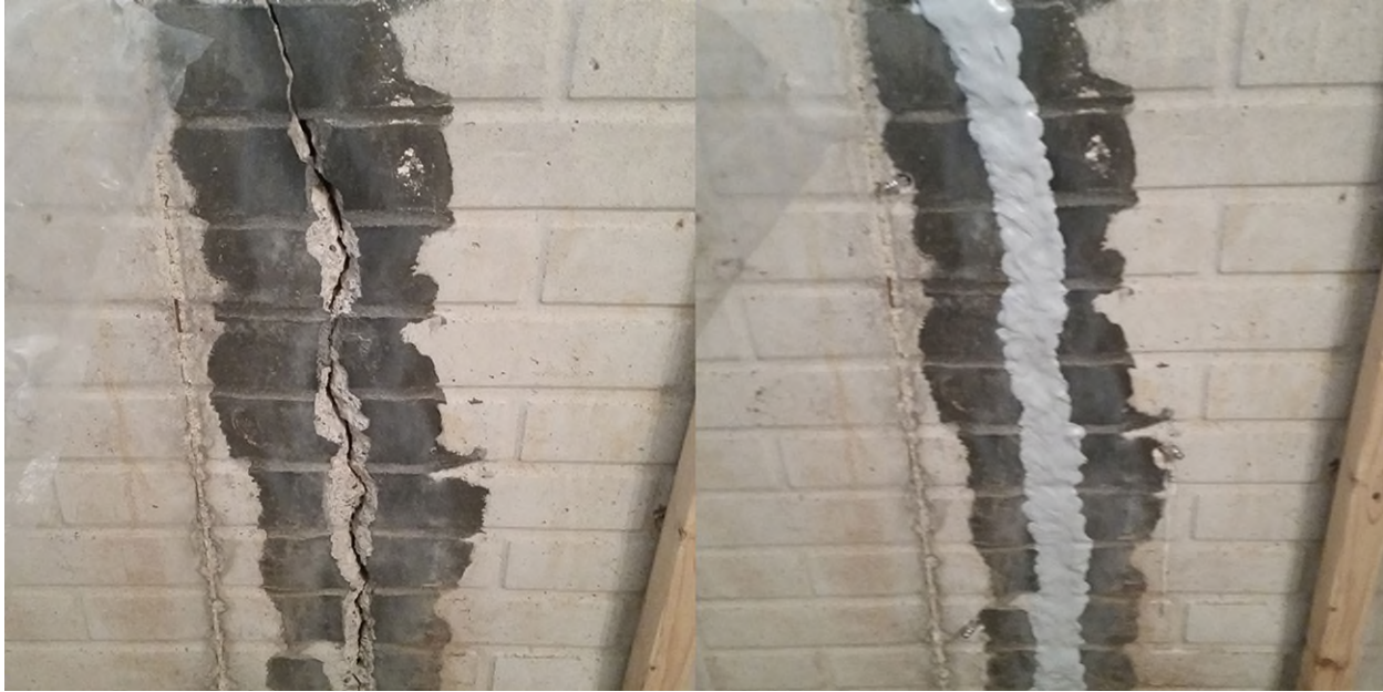
Figure 6. Waterproofing of a cracked basement wall (Absolutely Dry Basement Waterproofing, Inc, 2023)
