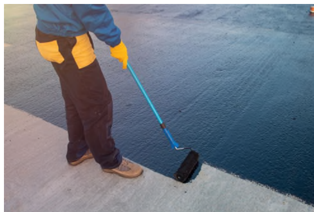
Figure 5. Waterproofing of Concrete Surface (Courtesy: ANDERSAL)
