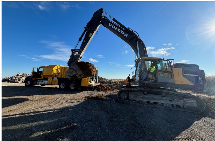
Figure 3.2 Soil excavation at Plattsmouth site
