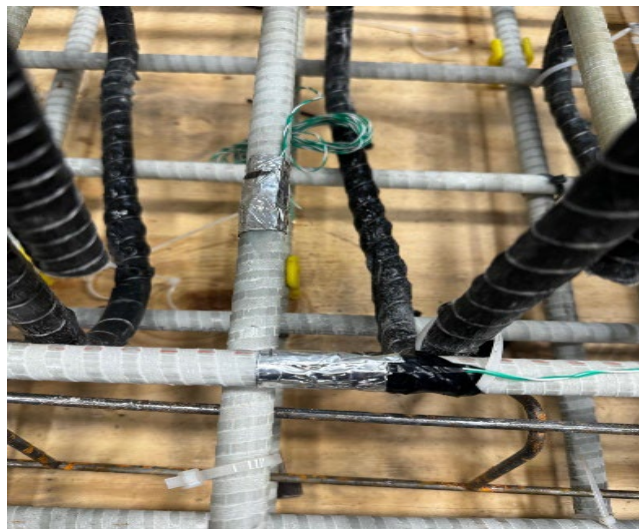
Figure 3.12 strain gauge installation
