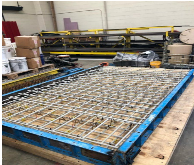
Figure 3.3 deck formwork/reinforcement
