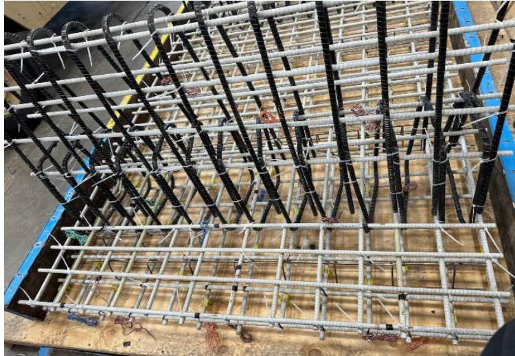
Figure 3.13 total number of strain gauge installation
