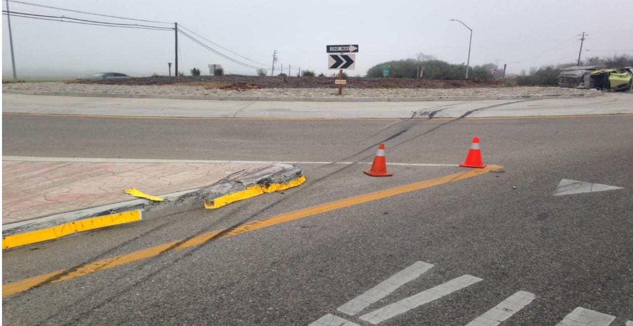
Figure 3.6: Example of a roundabout and splitter island incident. Image courtesy of Caltrans.
