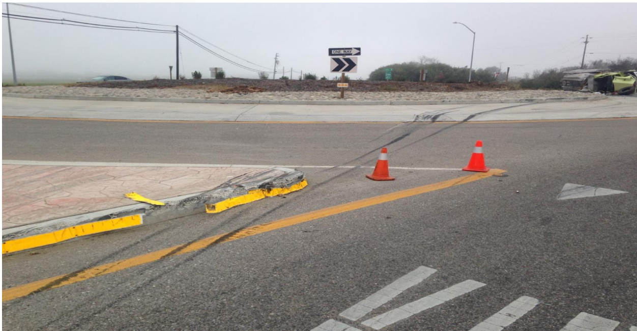
Figure A.10: Example of a roundabout and splitter island incident. Image courtesy of Caltrans.
