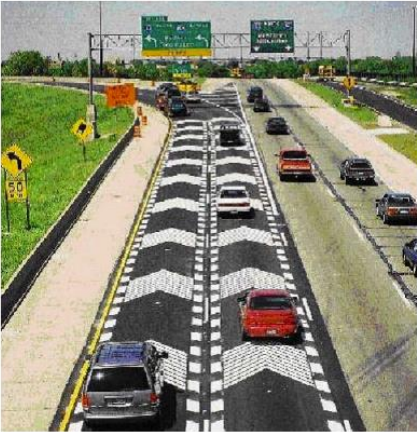
Source: Report on Passive Speed Control Devices, 2004
