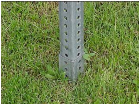
Figure E.11: Square tube breakaway post. Image courtesy of PennDOT [19].
