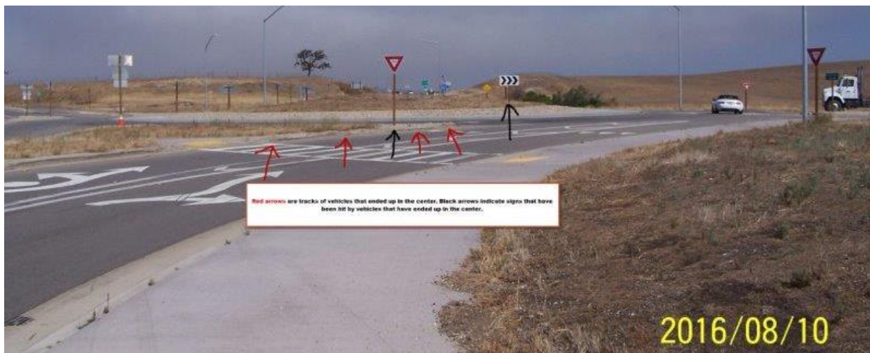
Figure A.7: Roundabout exposes maintenance workers to 360 degrees of upcoming traffic. Red arrows are tracks of vehicles that ended up in the center.
