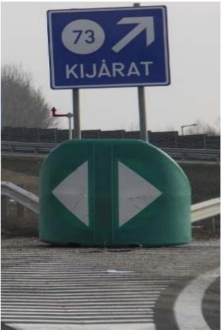
Impact attenuator with large retro-reflective bi-directional arrows
