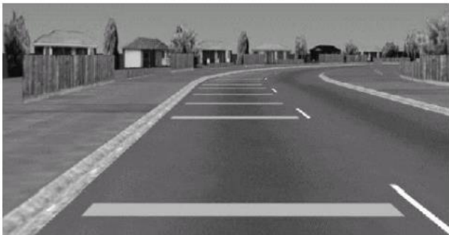
Source: Report on Passive Speed Control Devices, 2004
