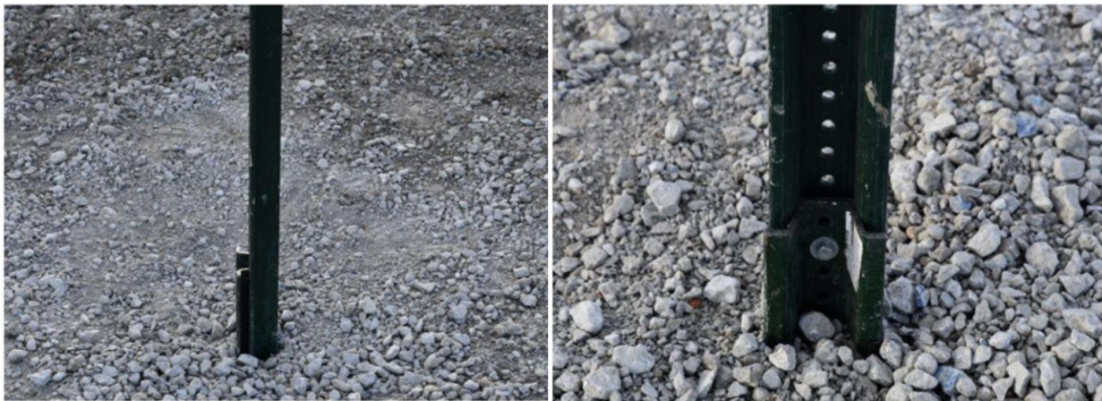
Figure E.10: U-channel post installation (page 25 of [18])
