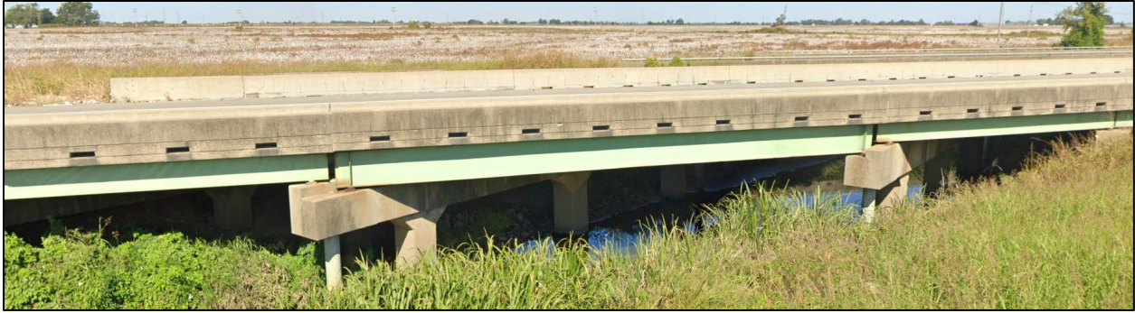
Figure 2.14 The elevation view (real image) of the L472 Bridge
