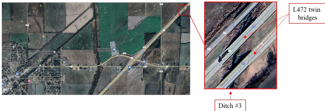
Figure 2.12 Satellite images of the L472 Bridge site
