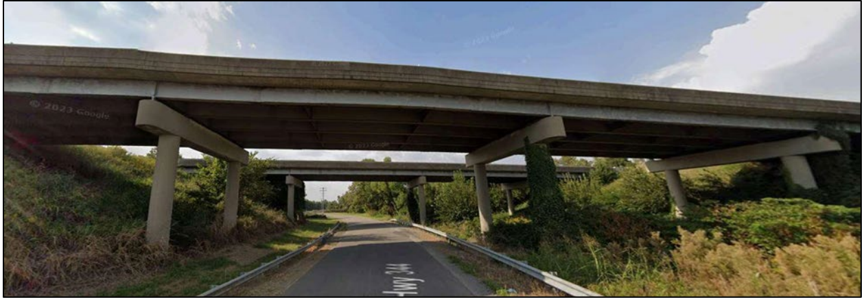
Figure 2.5 A1466 Twin Bridges (real image)
