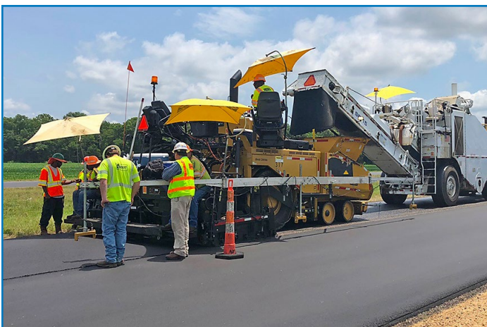
EDC-6 promoted asphalt overlay mixtures with materials and agents that reduce rutting, increase cracking resistance, and extend pavement life.
