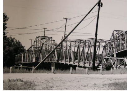
Figure 1.3 Utica Swing Bridge, 1906
