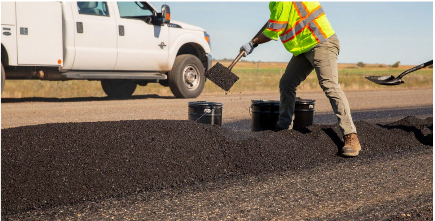
Figure 2. Photo of sampling location prior to the paver.
