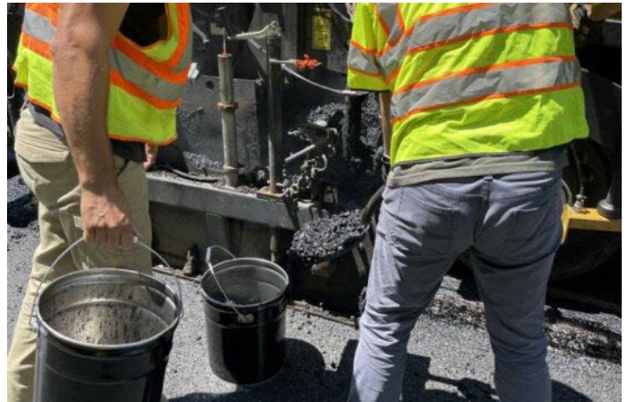
Figure 3. Photo of sampling location at the paver.
