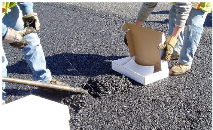
Figure 4. Photo of sampling location behind the paver.
