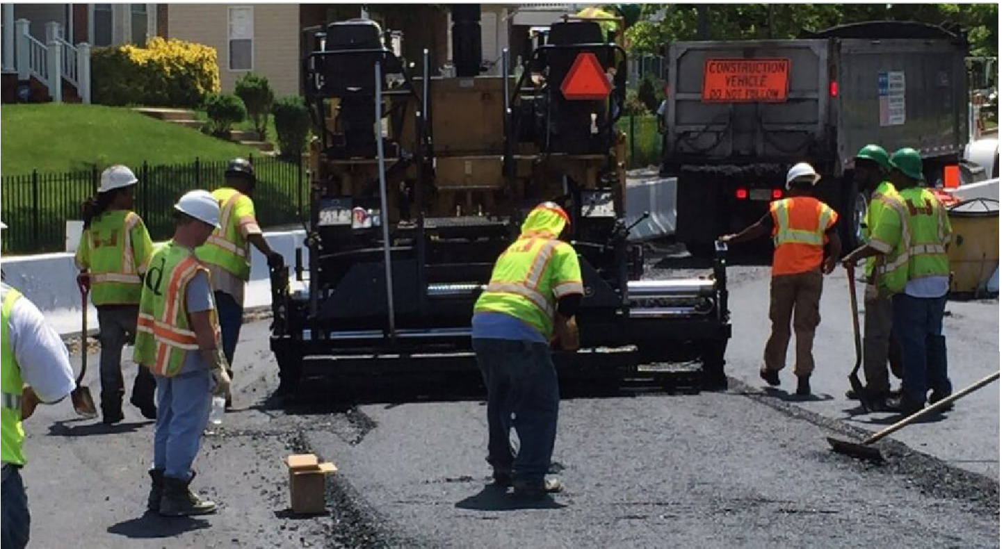
Figure 6. Photo. Asphalt sampling in the constructed mat behind the paver.
