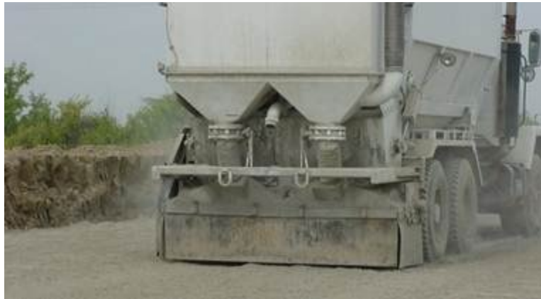
Figure 4 Dry Spreading Chemical Admixture on the Subgrade (from ODOT 2013)
