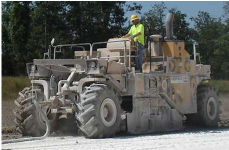
Figure 5 Large Rotary Mixer used for Chemical Stabilization (from ODOT 2013)
