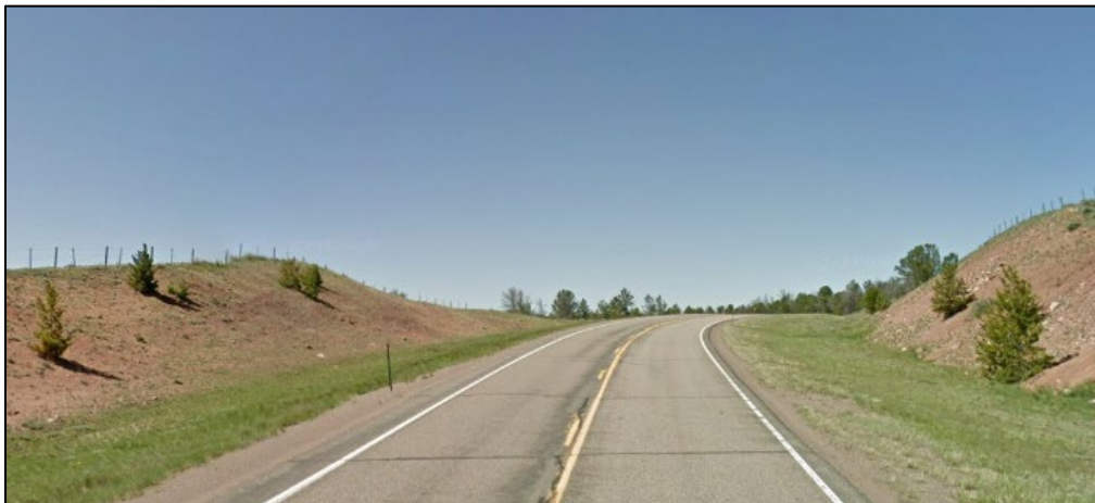
Figure 3.5 Section of Happy Jack Road with restricting sight distance. Source: Google L.L.C. (2021) (27)
