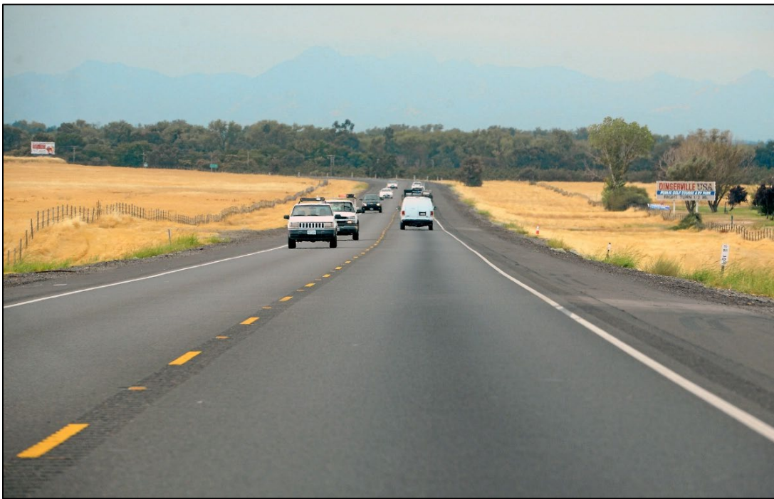
Figure 1.1 Two-lane highway. Source: (1)
