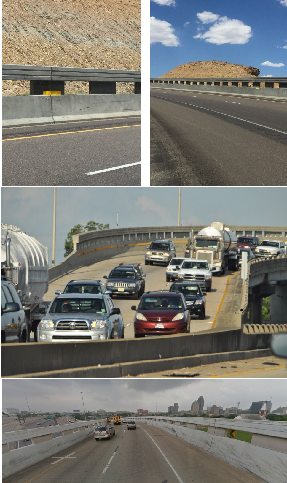
Figure 1.3 TL-6 Roman Wall Installations - Utah (top), Louisiana (middle), and Texas (bottom)
