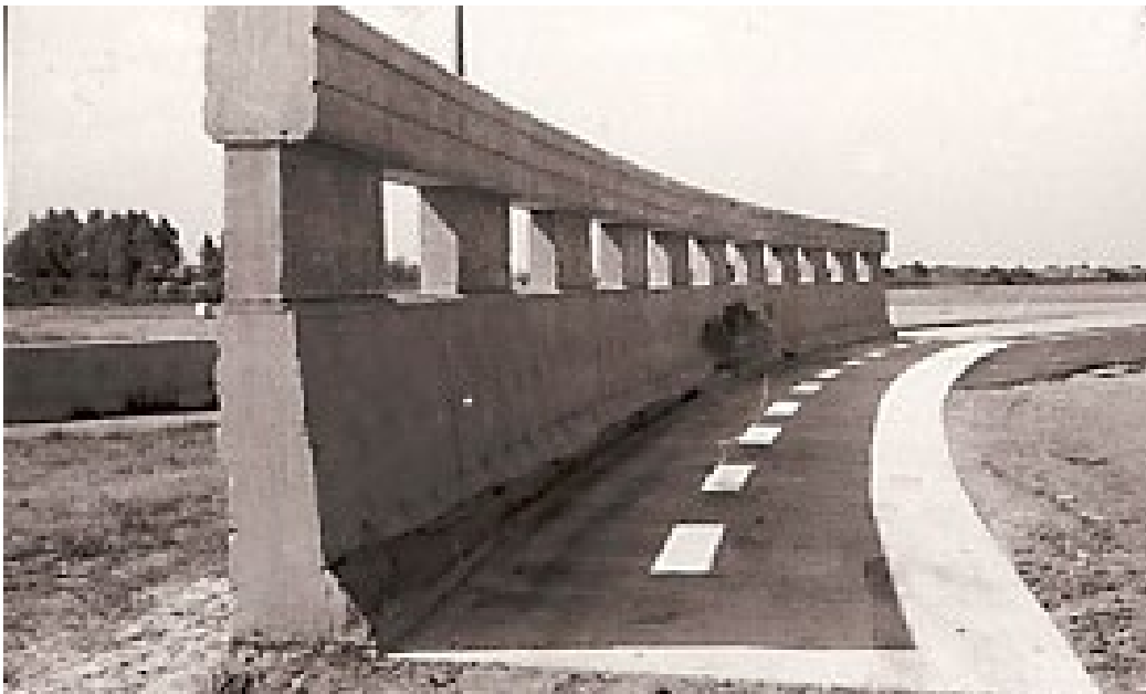
Figure 1.1 90-in. Tall, Combination Barrier System for Tractor-Tank Trailer Impact Events [4]
