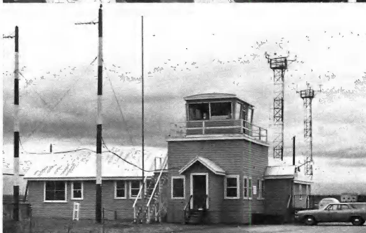
The Airway Facilities Sector Field Office at Galena is shared with the military.
