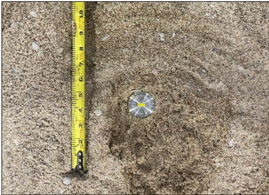
Figure 3.14 Pressure cell on compacted sand layer.
