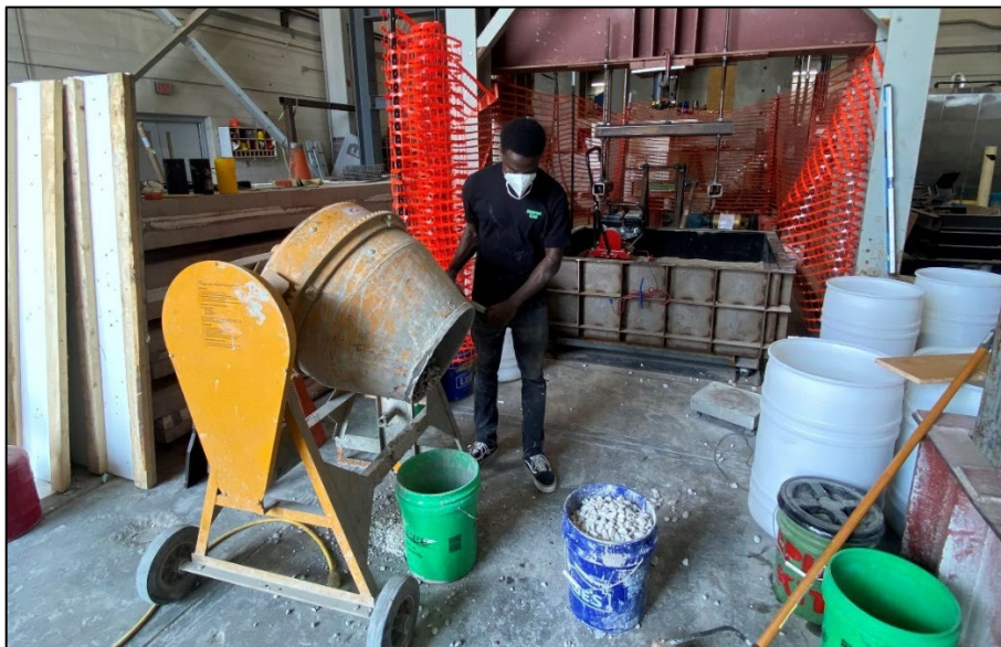
Figure 3.10 Aggregate mixing at OMC using concrete mixer.
