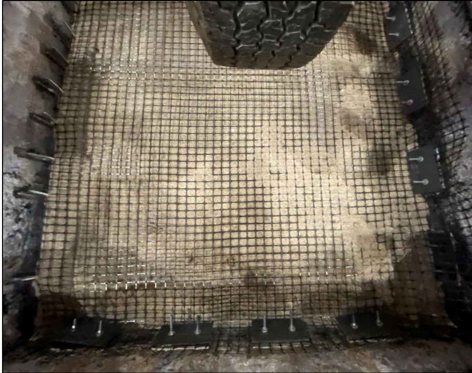
Figure 3.9 Installed geogrid on sand subgrade.
