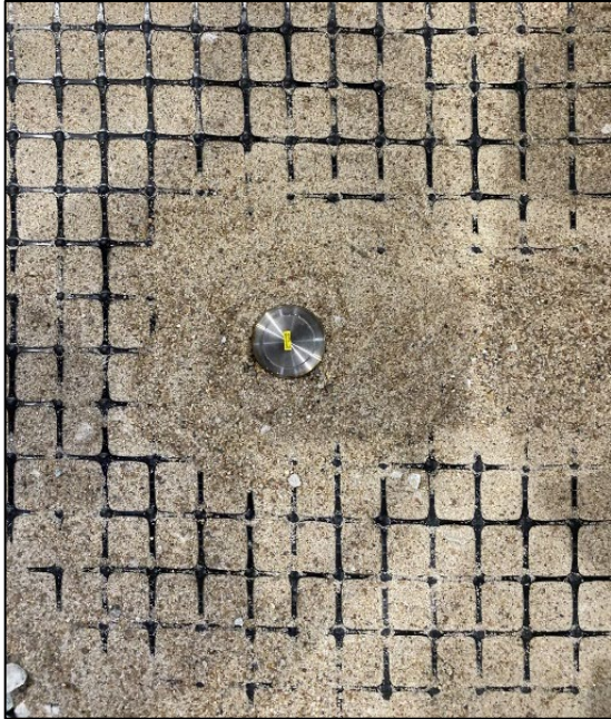
Figure 3.15 Pressure cell installed on top of geosynthetic location.
