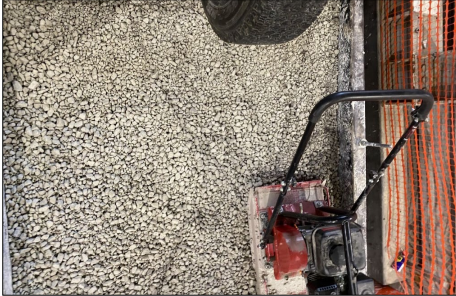
Figure 3.11 Compacted aggregate base course layer.
