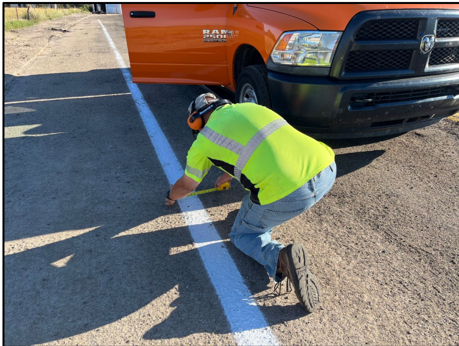
Figure 2.4: Confirmation of Lane Width During Manual Painting
