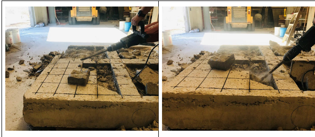
Figure 4.19 Removal of the discretized concrete pieces
