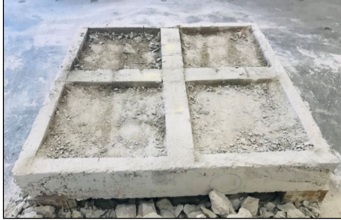
Figure 4.12 The concrete slab after jackhammer removal
