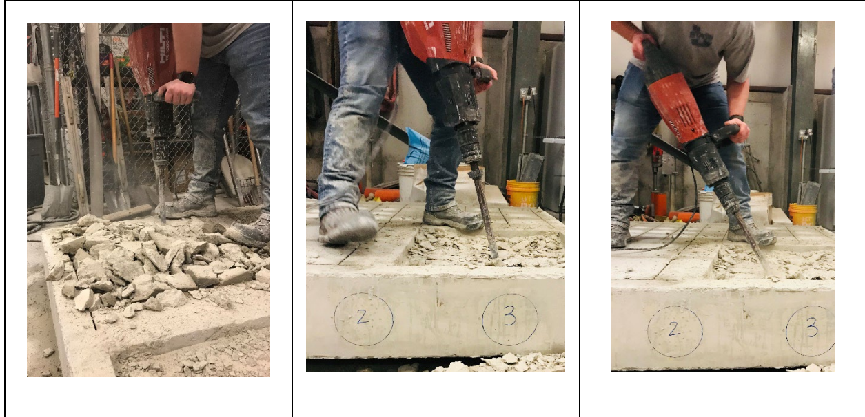
Figure 4.17 Examples of pull-off/impact angles of the jackhammer
