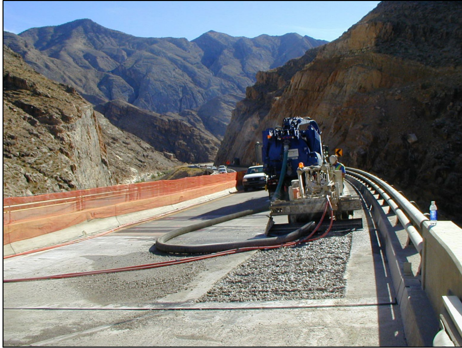
Figure 2.4 Hydro-demolition procedure
