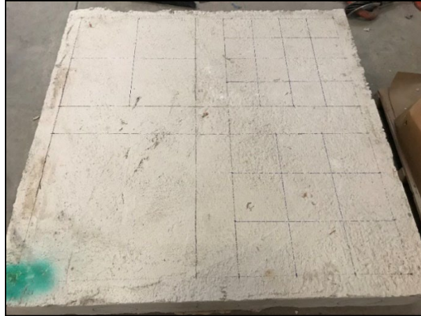
Figure 4.8 Preparation of the concrete slab before saw-cutting
