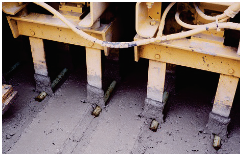
Figure 19. Typical dowel bar inserter (DBI) system (ACPA 2018).
