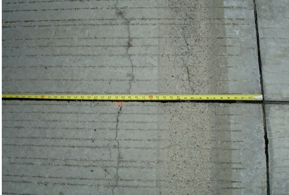
Figure 31. Restraint cracking at transverse joint after placement of new concrete shoulder in the next construction season.
