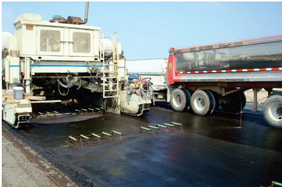
Figure 16. Illinois State Toll Highway Authority use of 5-dowel “mini-baskets” in each wheel path.
