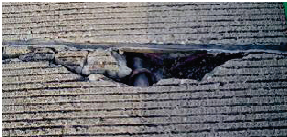
Figure 23. Photo of joint spalling caused by misaligned/mislocated dowel.
