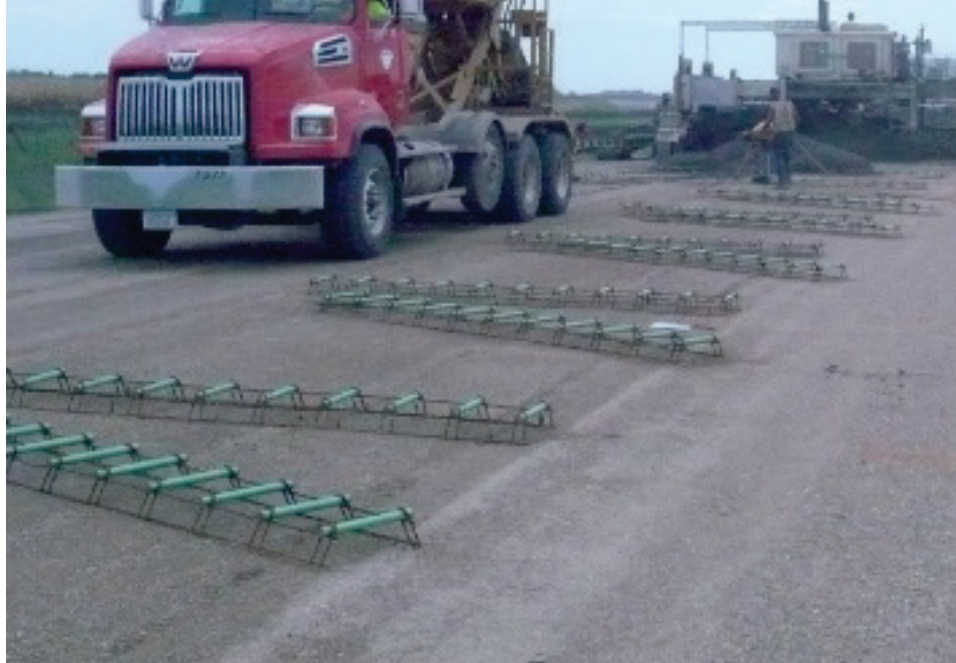
Figure 14. Use of 11-dowel baskets in Minnesota.
