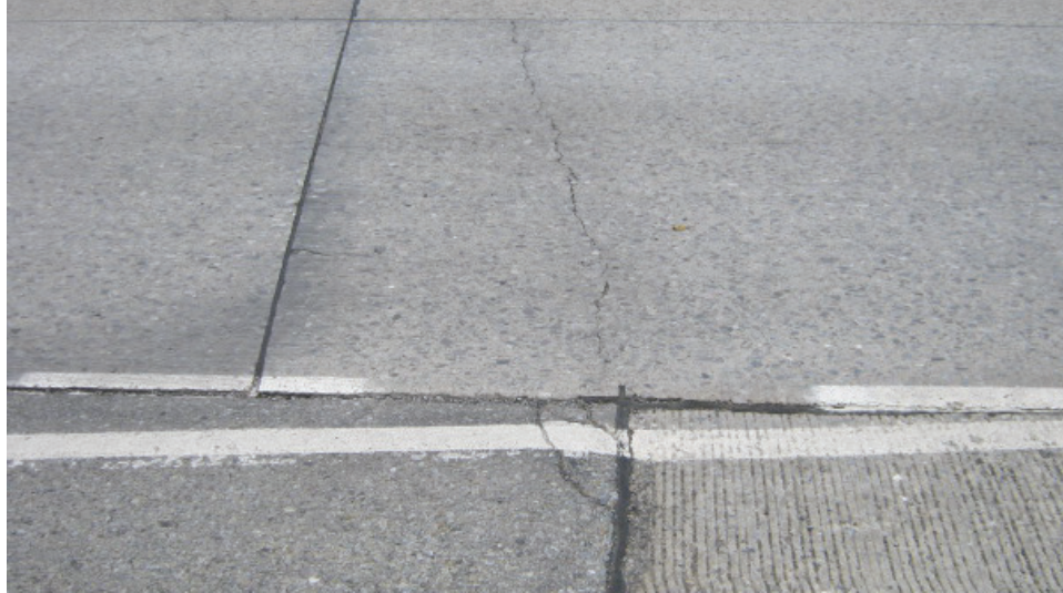
Figure 9. Propagation of crack due to misaligned transverse joints.
