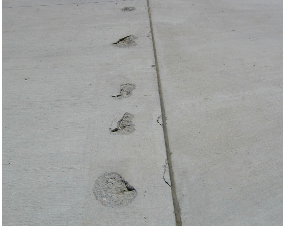
Figure 24. Misaligned dowels causing surface distress (Voigt and Ferrebee 2016).
