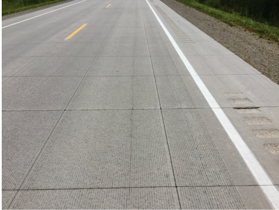
Figure 17. Photo of longitudinal cracking off ends of oversized tie bars in bonded concrete overlay of asphalt pavement in Iowa with widening (original pavement joint under longitudinal joint nearest stripe) – revised design calls for 1/2-in maximum tie bars in similar cases.
