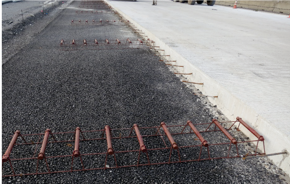
Figure 18. Dowel baskets on grade before paving.
