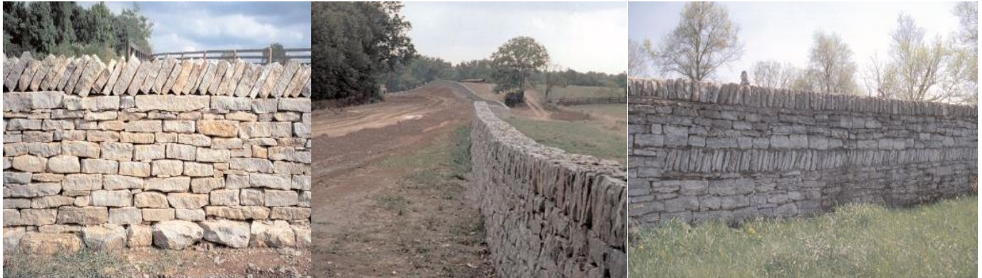
Instances of the Dry Stone fencing used along the Paris Pike Historic District. Credit: Paris-Lexington Road Design Team.
