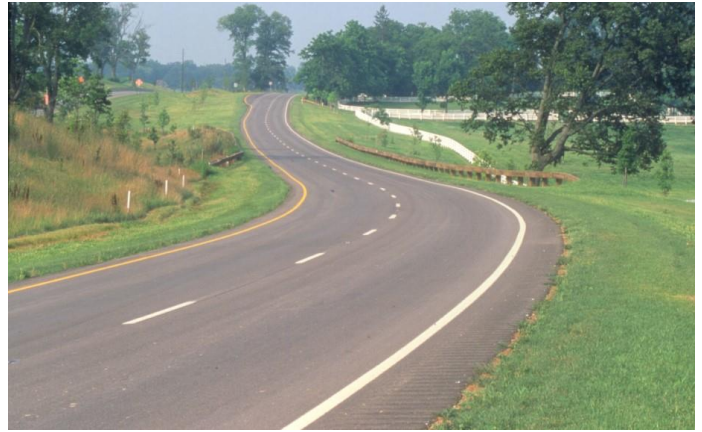
Timber guardrails separate Paris Pike from the many bur oaks that dot the surrounding woodland savannah landscape. Credit: Paris-Lexington Road Design Team.
