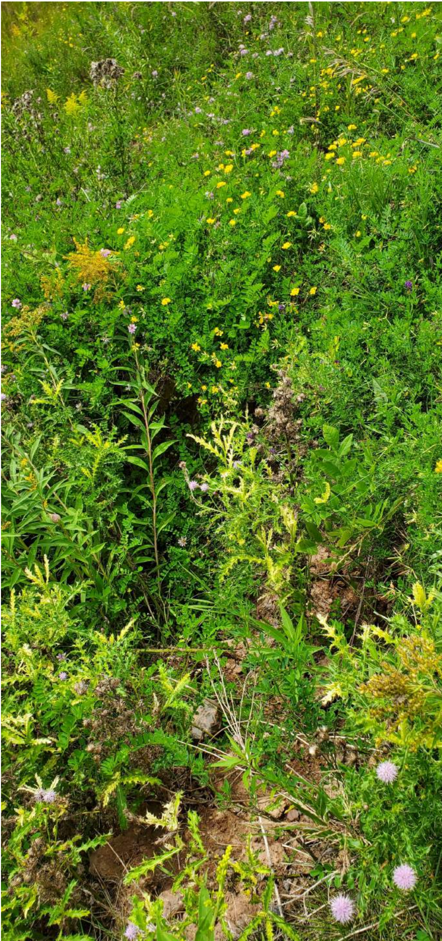
Figure 18. Older headscarp on the north side of MN210 at Site 4 near the channel created by the 2012 flood.
