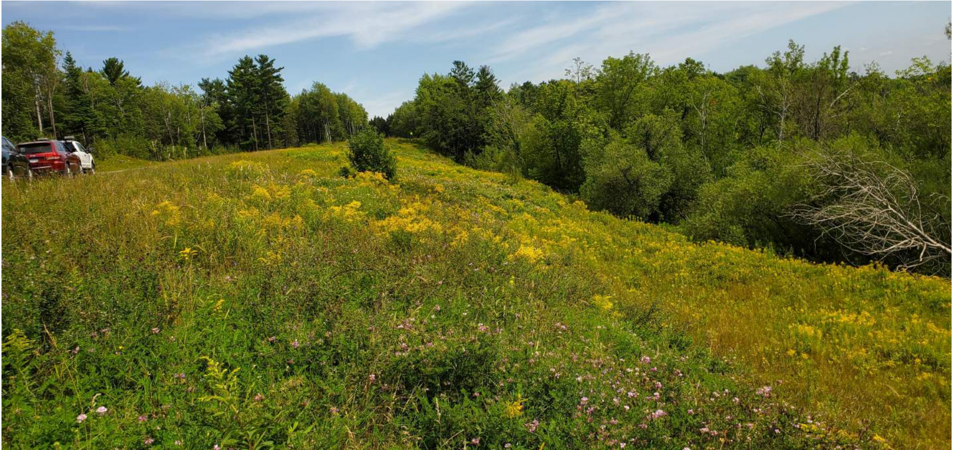
Figure 19. Graded slope on south side of MN210 at Site 4. Road was moved from the right side of the image to the left after the 2012 flood. St. Louis River is down the slope to the right.
