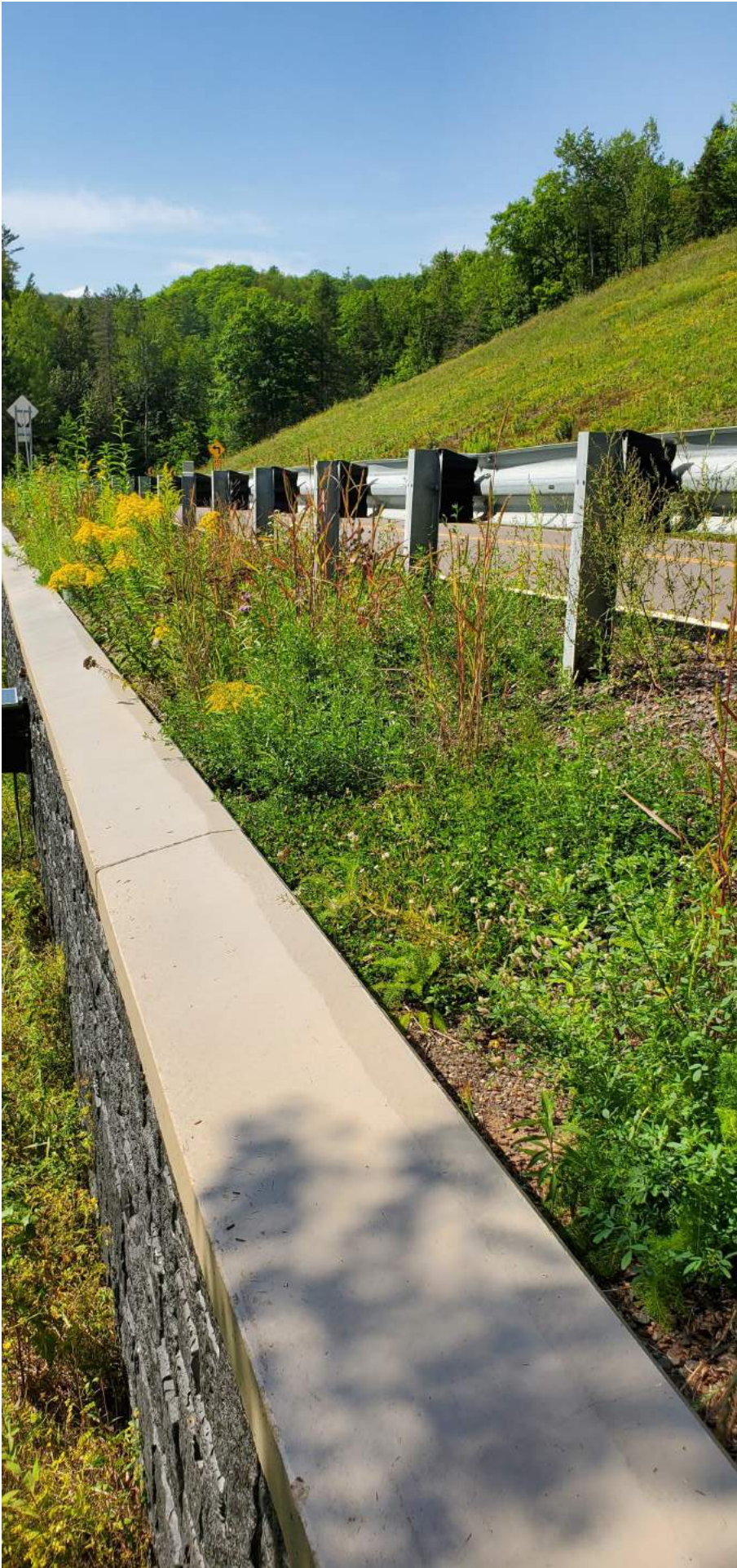
Figure 23. Retaining wall at Site 6.
