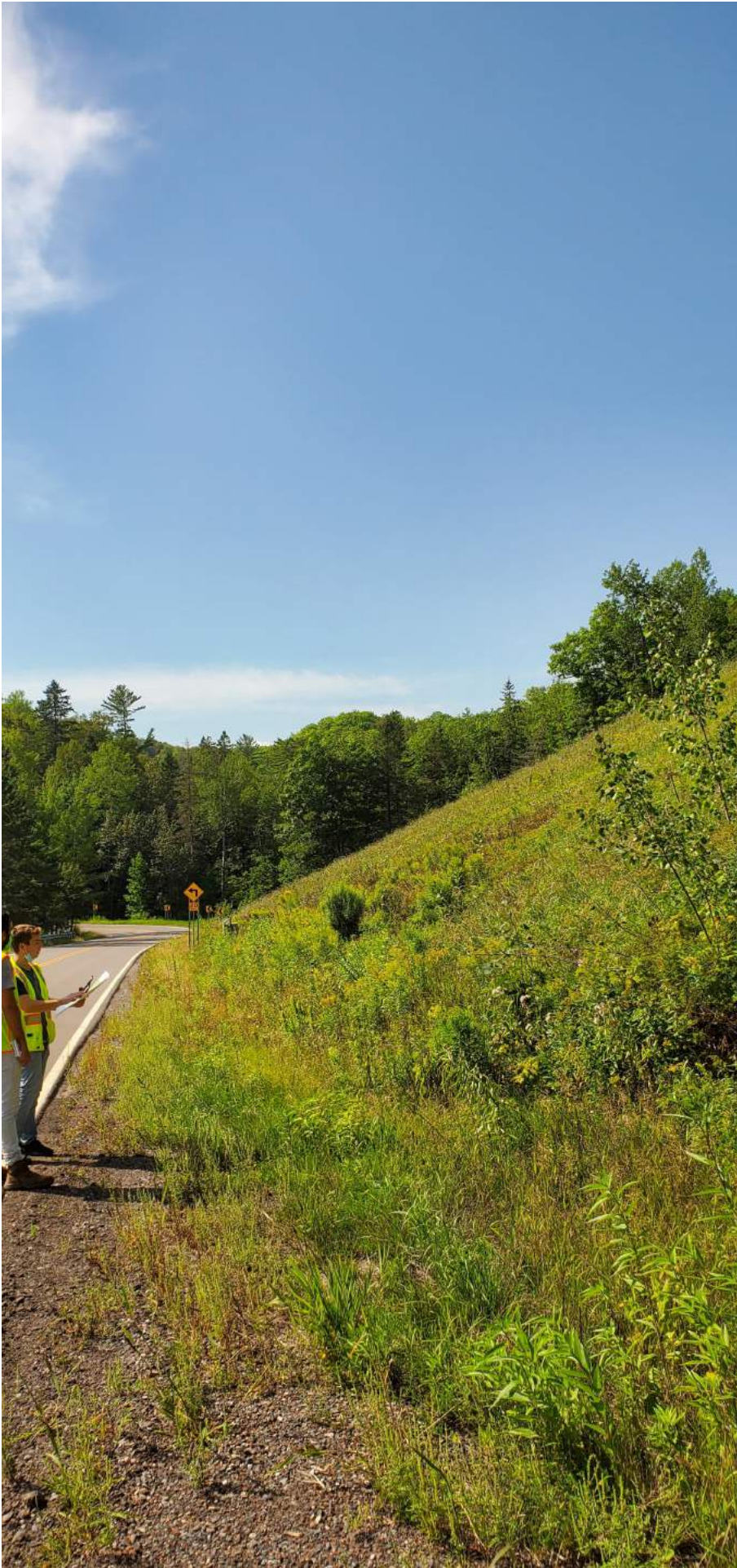
Figure 22. Graded slope at Site 6.
