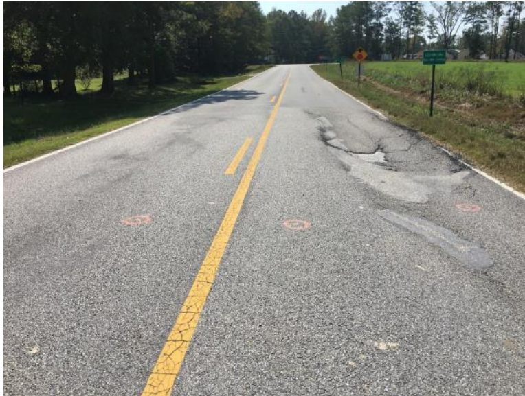
Figure 36. UTBWC in LR-159 five years after construction.
