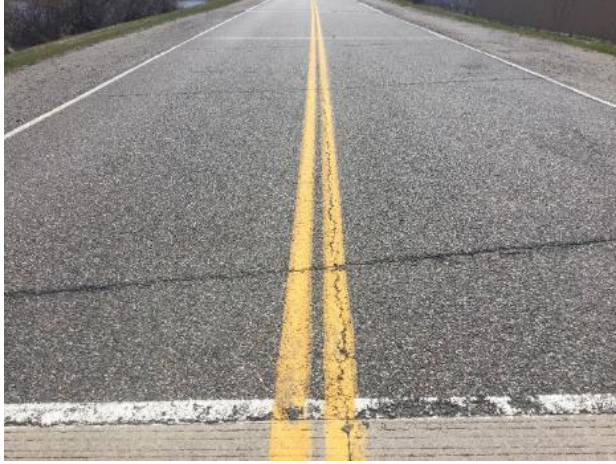
(a) OGFC over PCC (regular tack)
