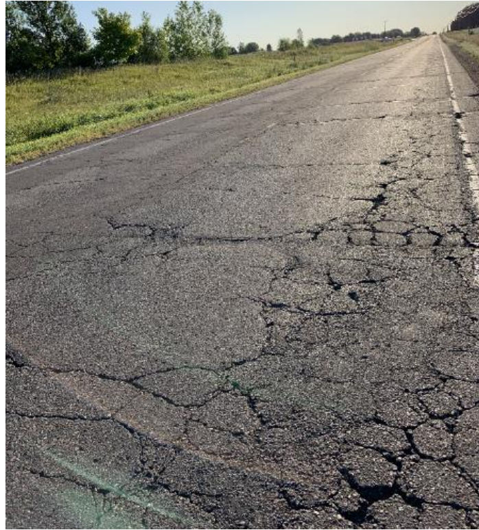
Figure 5. Overall pavement condition of 70 th Street.
