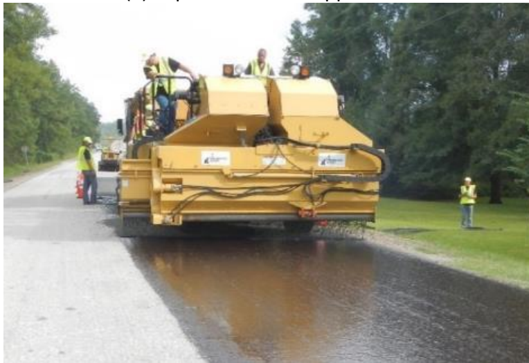
(b) Aggregate application
