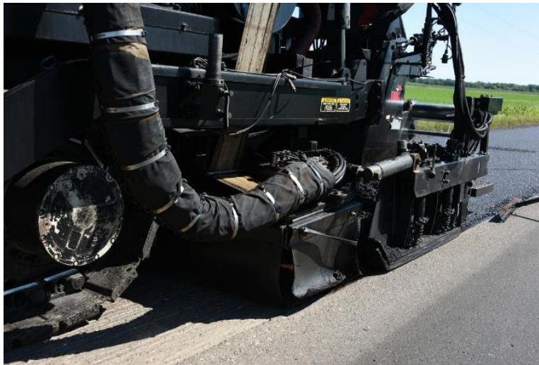
Figure 34. UTBWC application with spray paver (27).
