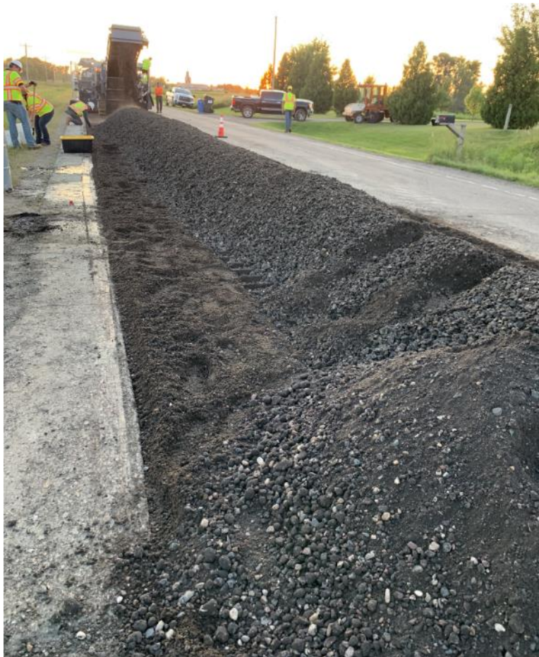
Figure 47. Reclaimed material in FDR section.
