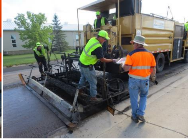
(b) Pan assembly handed to operator
