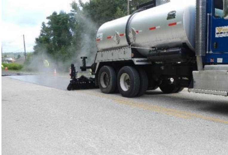
(a) Asphalt emulsion application
