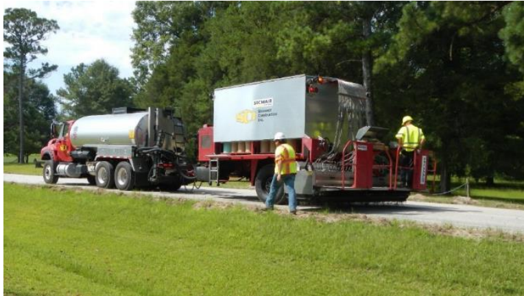
Figure 17. Fibermat® installation.
