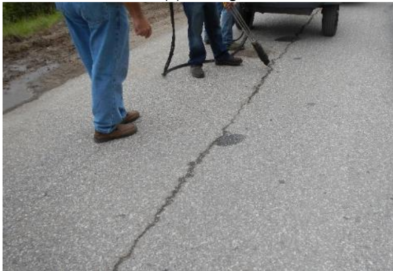
(b) Compressed air with a heat lance
