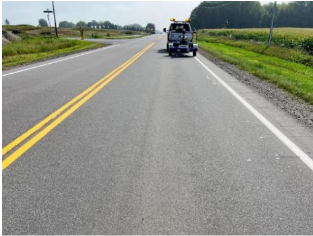
(a) CCPR – foamed asphalt
