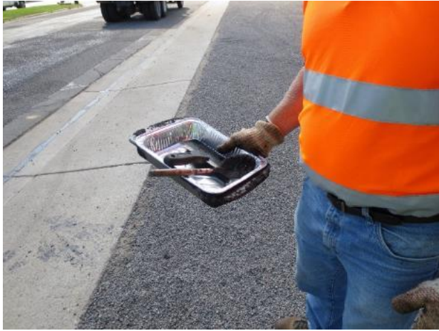
(a) Pan assembly and mixing tools
