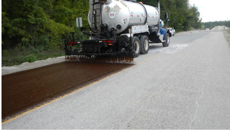
Figure 13. Fog seal application.
