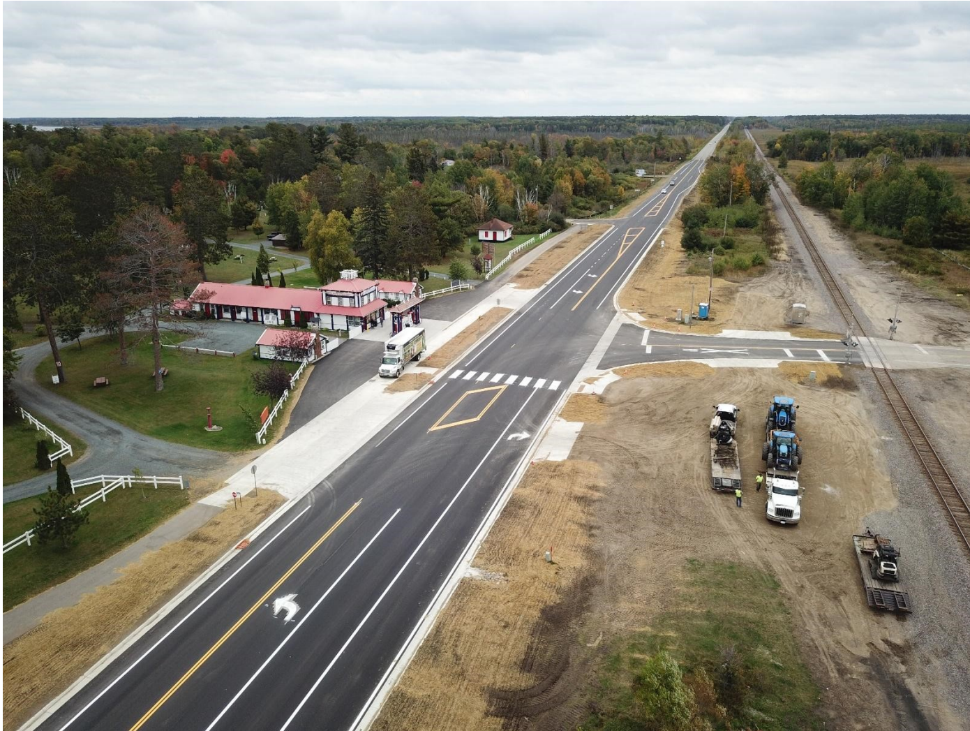
Figure 4.9 Bena: Hwy 2 and 1st Ave countermeasures (2023, from west).
