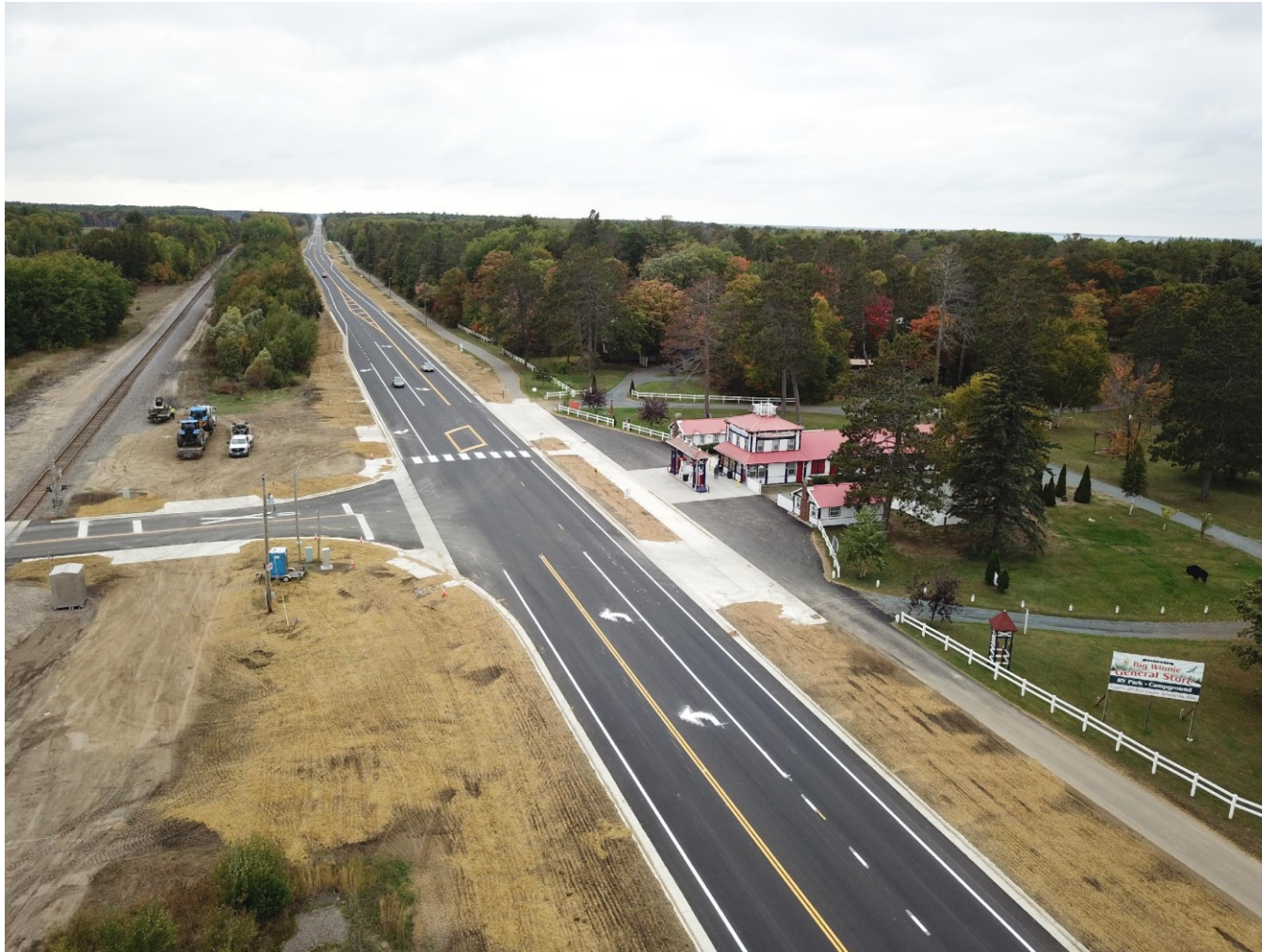
Figure 4.10 Bena: Hwy 2 and 1st Avenue countermeasures (2023, from east).
