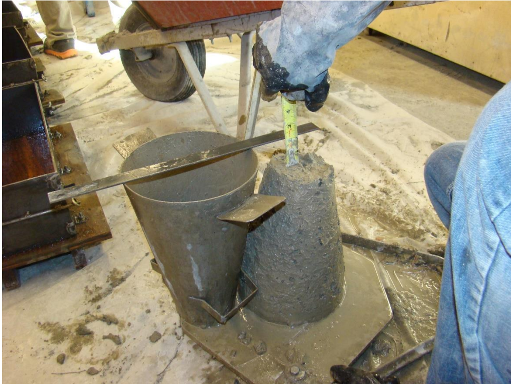
Figure 8-15: Measurement of the concrete slump, according to ASTM C143
