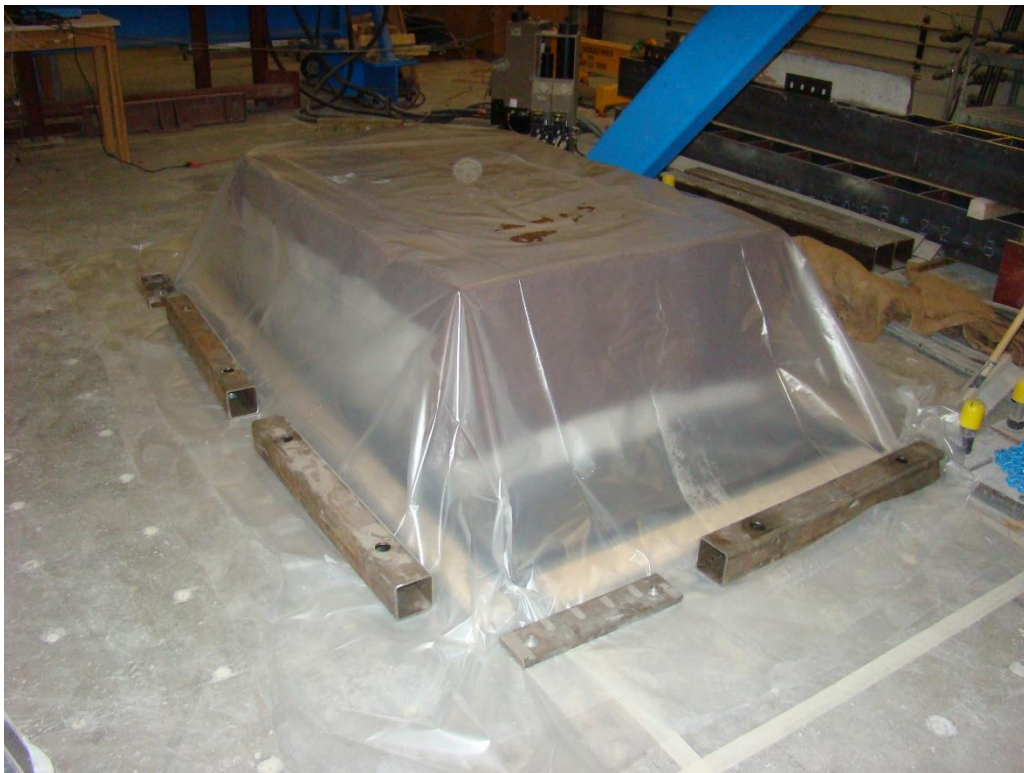
Figure 8-14: Plastic sheet placed over the top of the wet burlap to seal in the moisture
