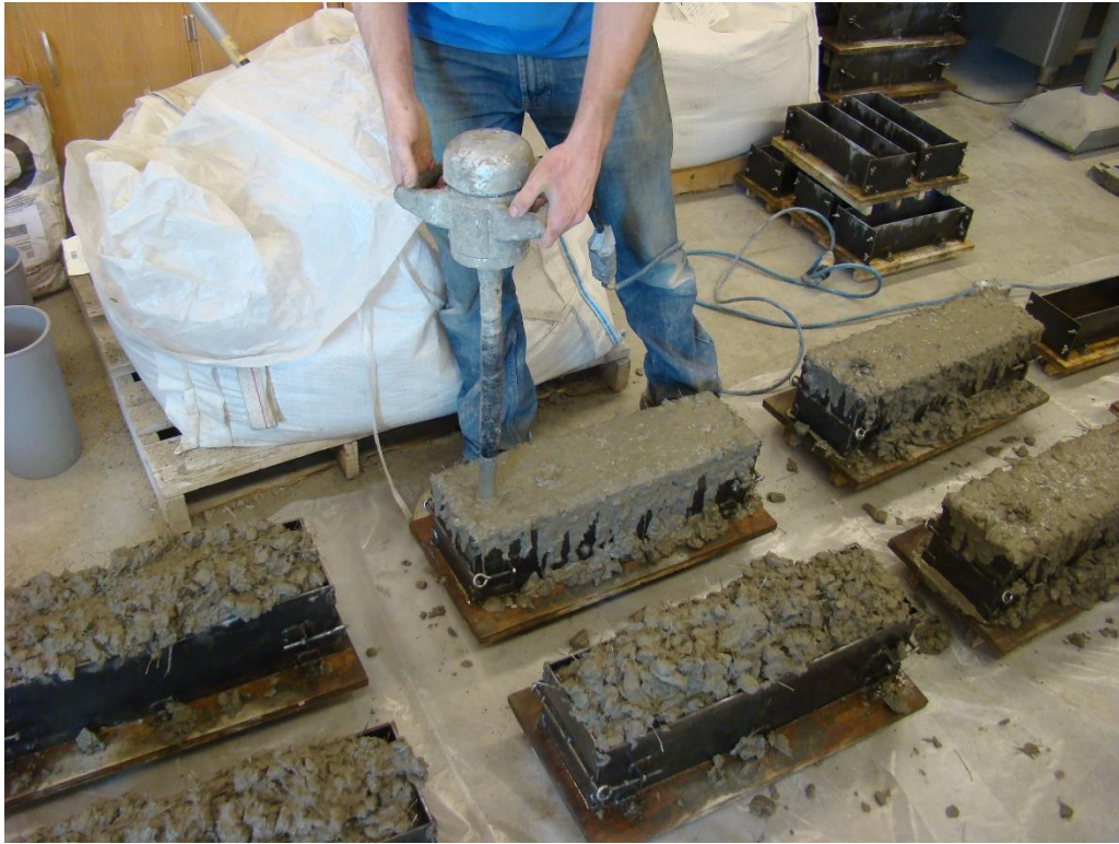
Figure 8-10: Hand-held spud vibrator in use
