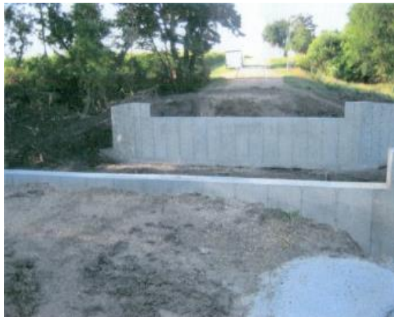
Figure 3-1u: Completed abutments.
