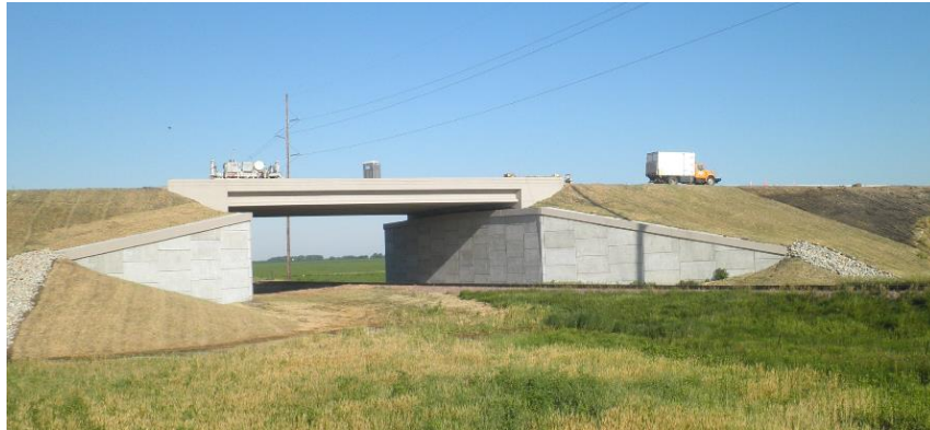
Mechanically Stabilized Earth (MSE) Wall
