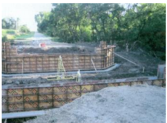
Figure 3-1r: Abutment wall formwork.
