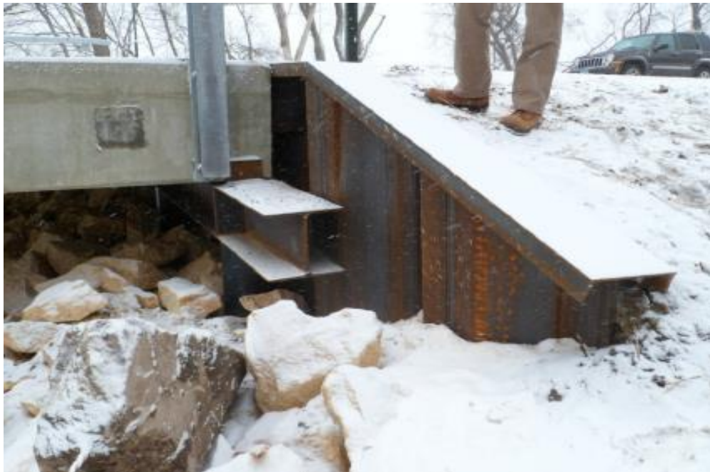
Figure 2-10: Sheet pile abutment (MnDOT, 2012)
