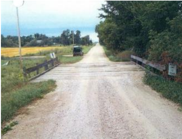
Figure 3-1a: Looking north prior to replacement.
