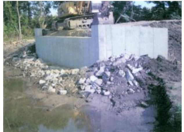
Figure 3-1v: Abutment backfill and riprap
