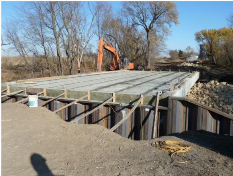
Sheet Pile Abutment
