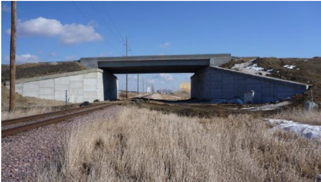
Figure 2-9: Mechanically Stabilized Earth (MSE) Walls (MnDOT, 2012)
