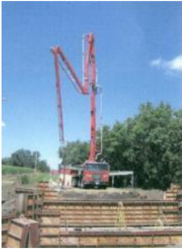
Figure 3-1s: Placement of abutment wall concrete.
