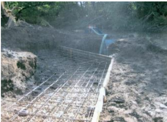
Figure 3-1o: Abutment footing reinforcement.
