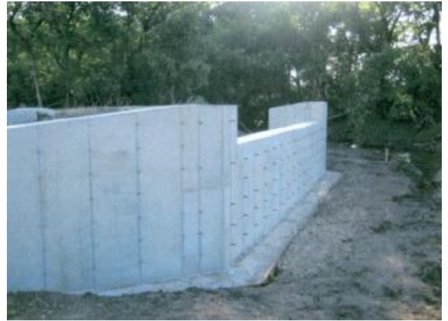
Figure 3-1t: Abutment backfill and riprap placement.
