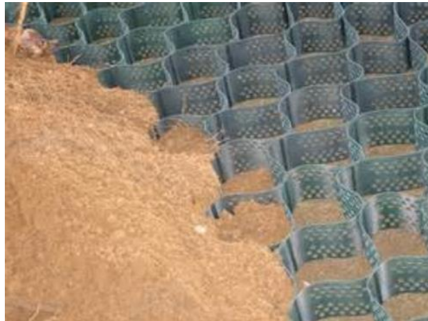
Figure 2-13: Cellular Confinement system (CCS) (Cell-Tek, 2010).
