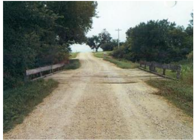
Figure 3-1b: Looking south prior to replacement.
