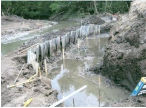
Figure 3-1m: Preparing site for abutment construction.
