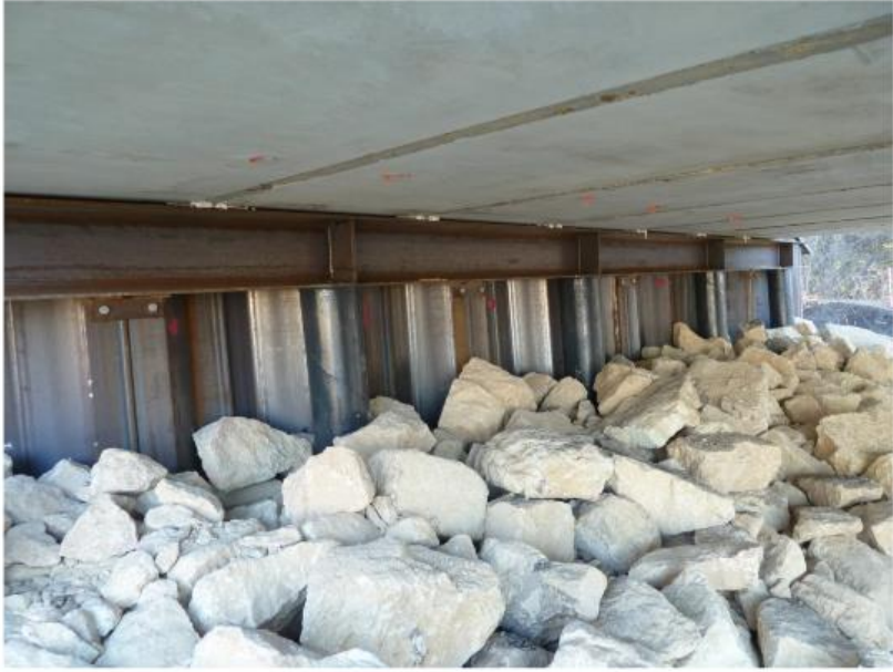
Sheet Pile Abutment
