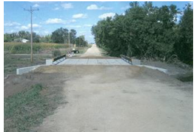
Figure 3-1x: Grade restored and railings installed. Project complete.
