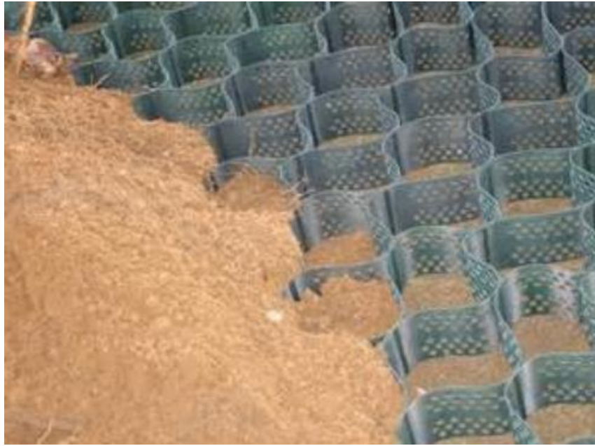
Cellular Confinement System (Cell-Tek, 2010).
