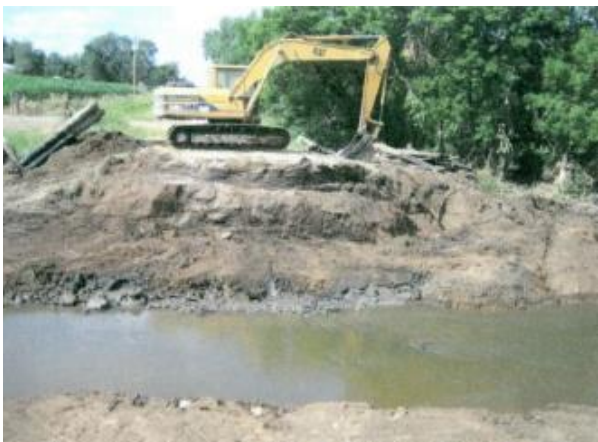
Figure 3-1k: Preparing site for abutment construction.
