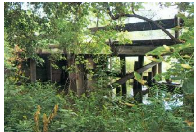
Figure 3-1d: Looking west prior to replacement.
