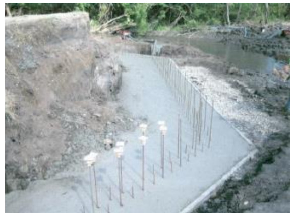
Figure 3-1p: Concrete placement with abutment reinforcement.
