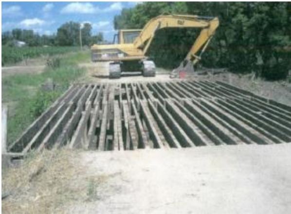
Figure 3-1i: Selective bridge demolition.
