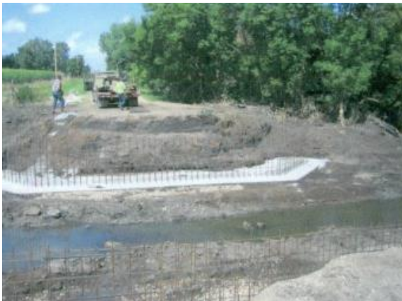
Figure 3-1q: Abutment wall reinforcement.
