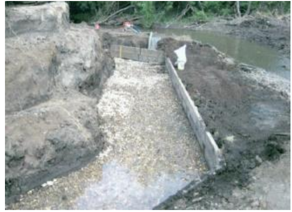
Figure 3-1n: Gravel placement prior to installation of reinforcing.
