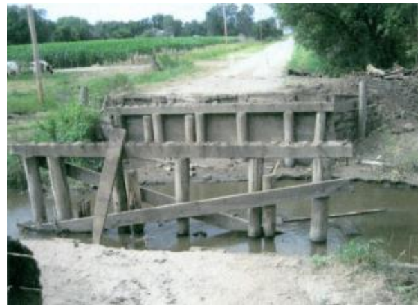
Figure 3-1j: Selective bridge Demolition.
