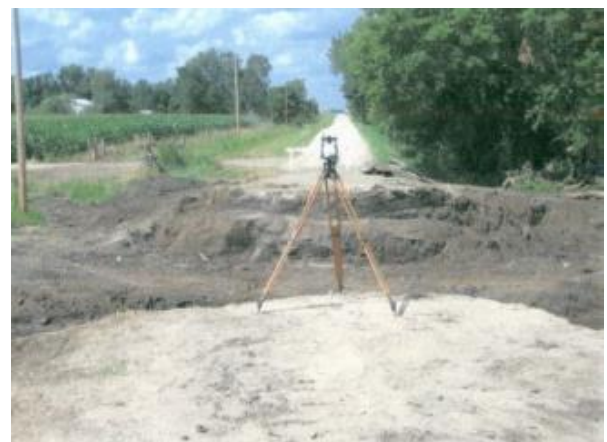
Figure 3-1l: Preparing site for abutment construction.
