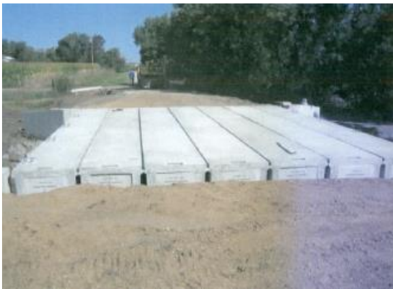
Figure 3-1w: Placement of adjacent box slabs.
