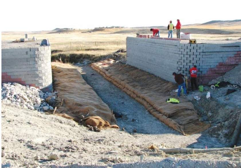
Geosynthetic Reinforced Soil (GRS) Abutment
