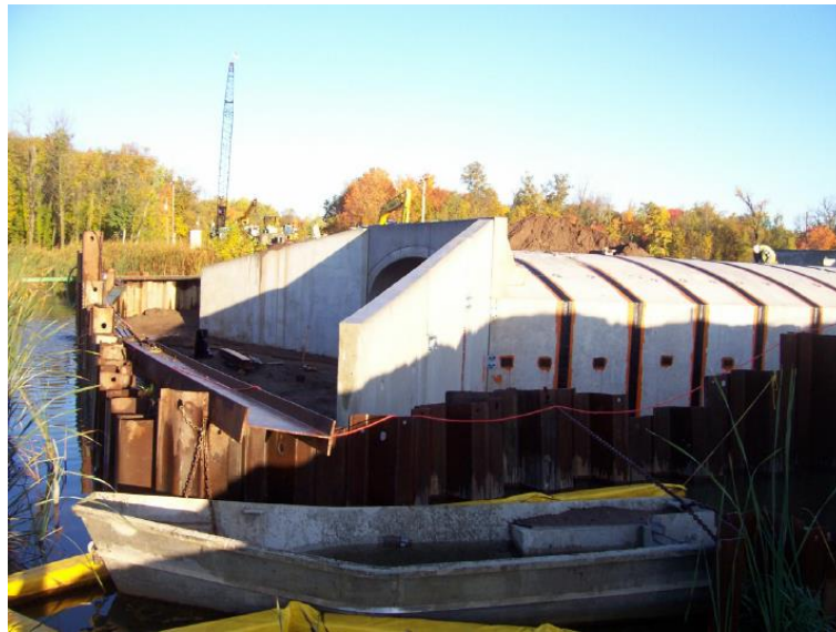
Figure 2-14: Precast Large Box Culvert (MnDOT, 2012)
