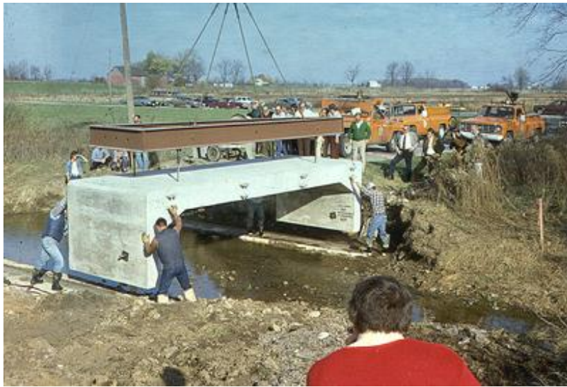
Figure 2-15: Three-sided frame (Ohio DOT, 2015)
