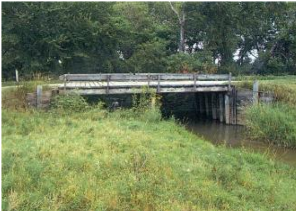
Figure 3-1c: Looking east prior to replacement.
