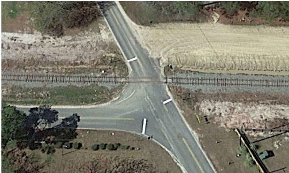
Figure 29: Satellite imagery showing crossing 732405Y
