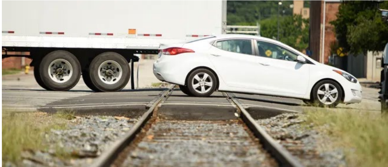
Figure 2: A humped high-profile grade crossing being negotiated by a passenger vehicle
