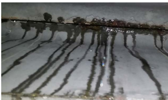
(a) Water Seepage through the Joint
