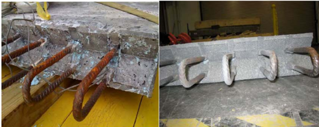
Figure I.5-1 U Bars at Joint
