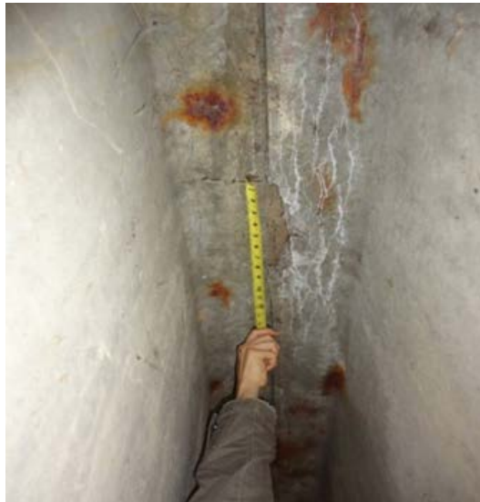
Figure 2-3: Concrete Deterioration in the Deck Overhang of a Double Tee Bridge
