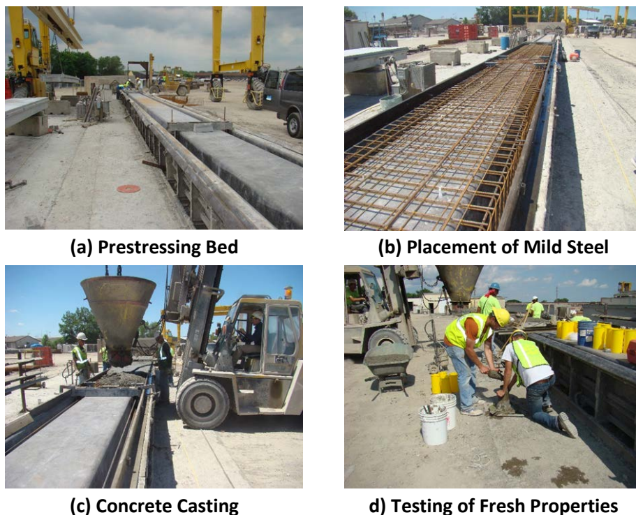
Figure 7-8: Fabrication of the Girders for the “Conventional” Specimen
