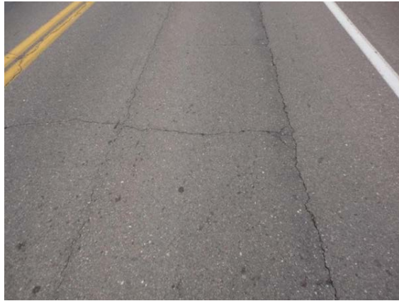
Figure 2-2: Reflective Cracking of the Asphalt Overlay
