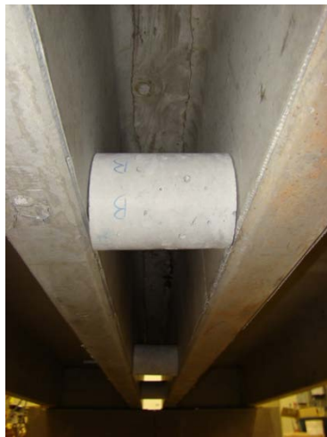
Figure 7-14: Restraining Diaphragm in Place
