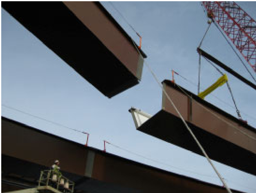
Steel Tub Girder Placement
