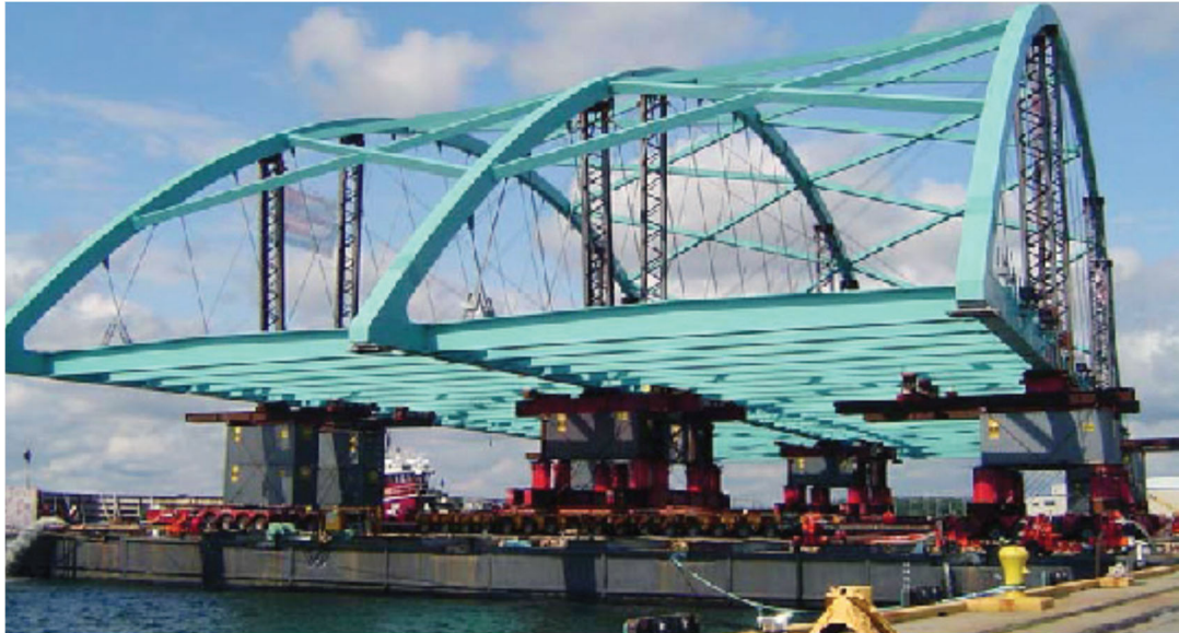
Replacement of Truss Span without Deck (Barge Use)
