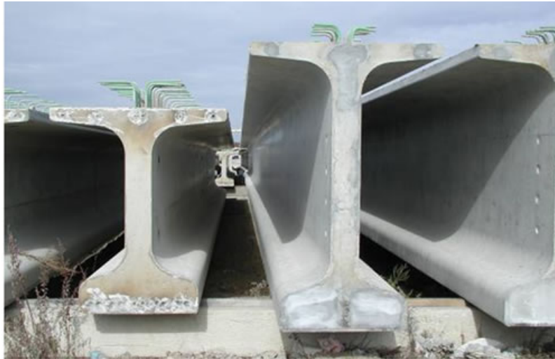
Precast Bulb-T Girders
