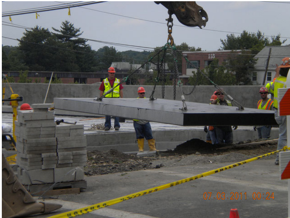
Precast Approach Slab Installation
