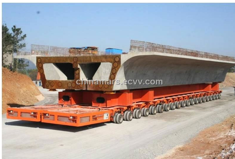
Self-Propelled Modular Transporter Carrying a Bridge Deck
