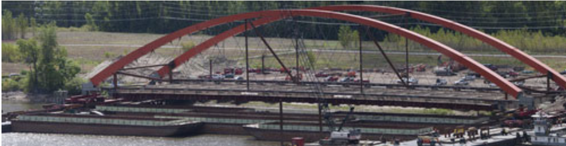
Hastings Arch Bridge with Deck Move (Barge Use) http://www.hastingsstargazette.com/event/photogallery/id/57/ Accessed 23 Oct 2012
