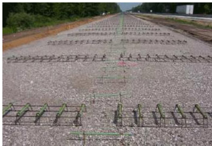
Figure 5-1: Tie Bars prior to Placing Concrete (Perera, Kohn, & Tayabji, 2005)
