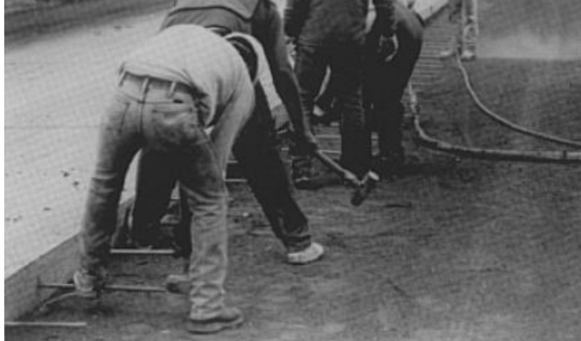
Figure 5-2: Installation of Drilled-in Tie Bars (South Dakota DOT, 2016)
