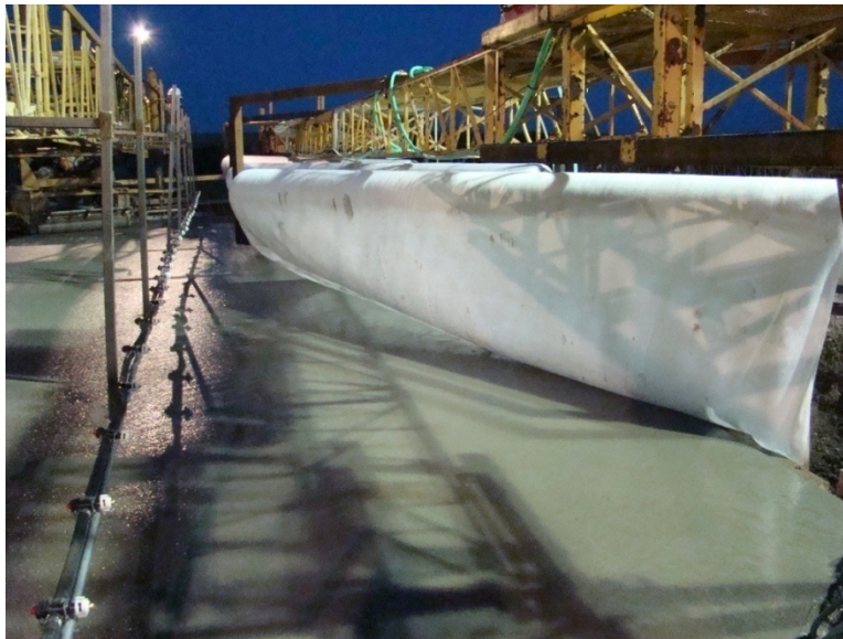
Fig. 8.27 Concrete Fogger Set Up for the LC-HPC Deck in Brule County
