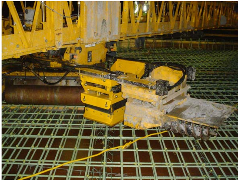
Fig. 8.18 Rotating Drums and Skewed Augur on the Finishing Machine
