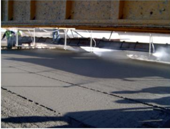
Fig 8.8 Finishing of Concrete
