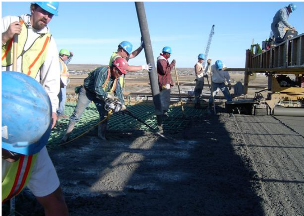
Fig. 8.7 Concrete Placement and Consolidation
