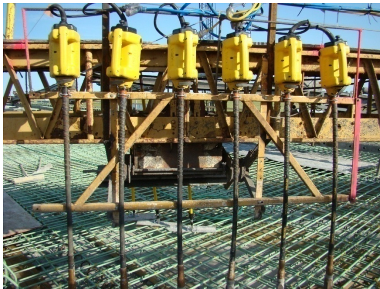
Fig. 8.26 Gang Vibrator Set Up for the LC-HPC Deck in Brule County
