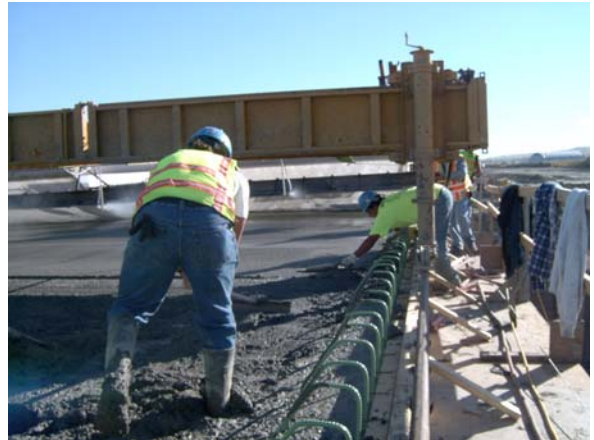
Fig 8.8 Finishing of Concrete
