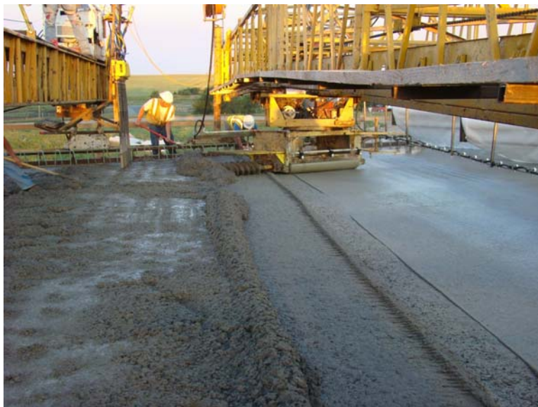
Fig. 8.25 Excess Concrete Deposit at the LC-HPC Deck in Brule County
