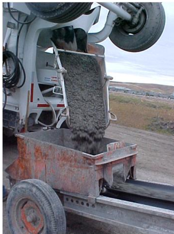
Fig. 8.11 Consistency of Concrete at the Back of the Truck
