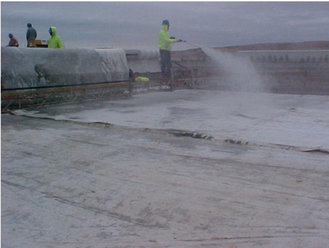
Fig. 8.17 Curing Blankets in Place and Being Water Soaked
