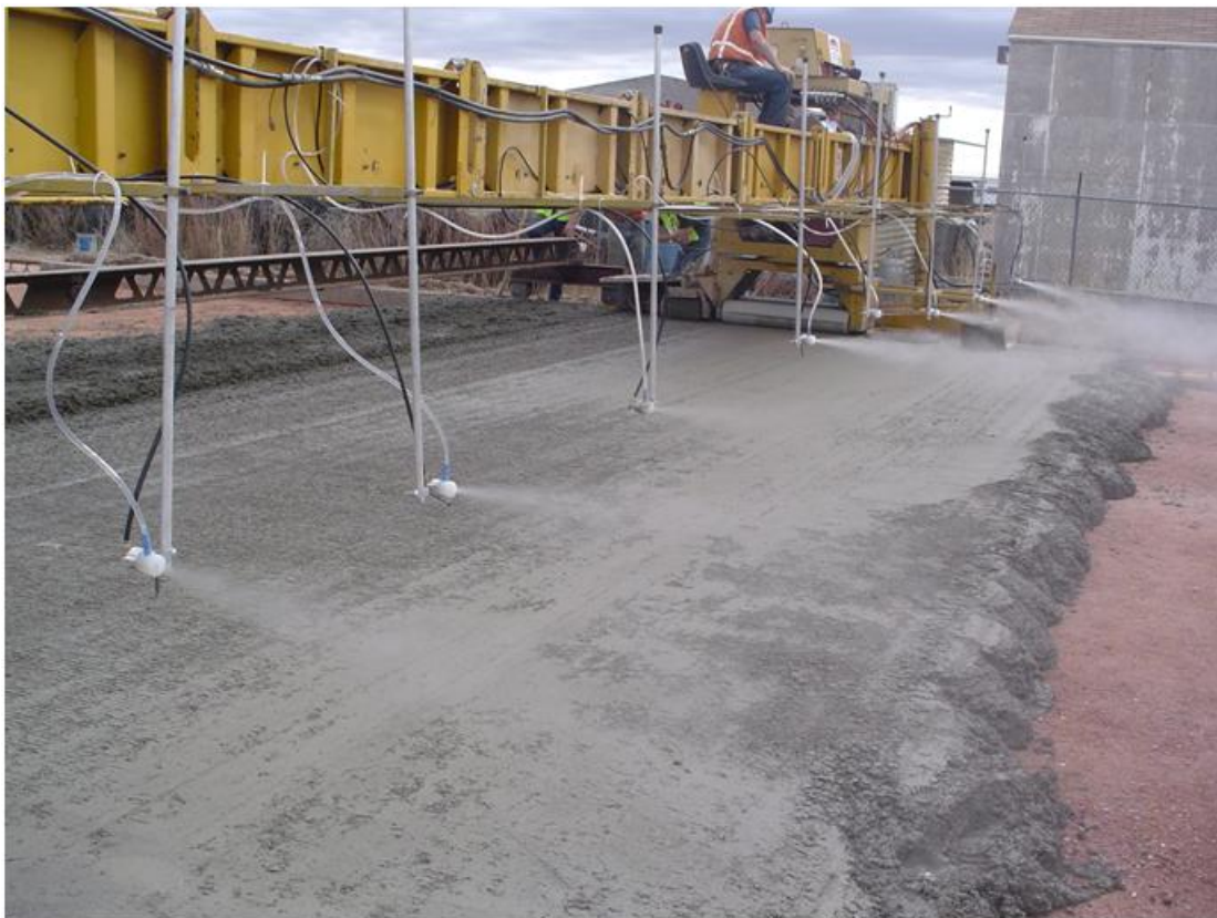
Fig. 8.4 Excessive Fogging Caused Puddles of Water over Wet Concrete
