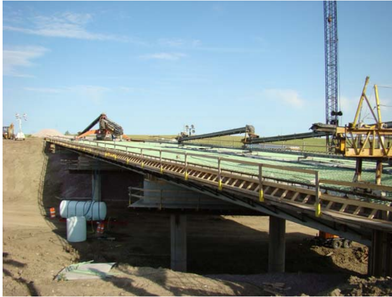
Fig. 8.24 Conveyor Belt Set Up for the LC-HPC Deck in Brule County
