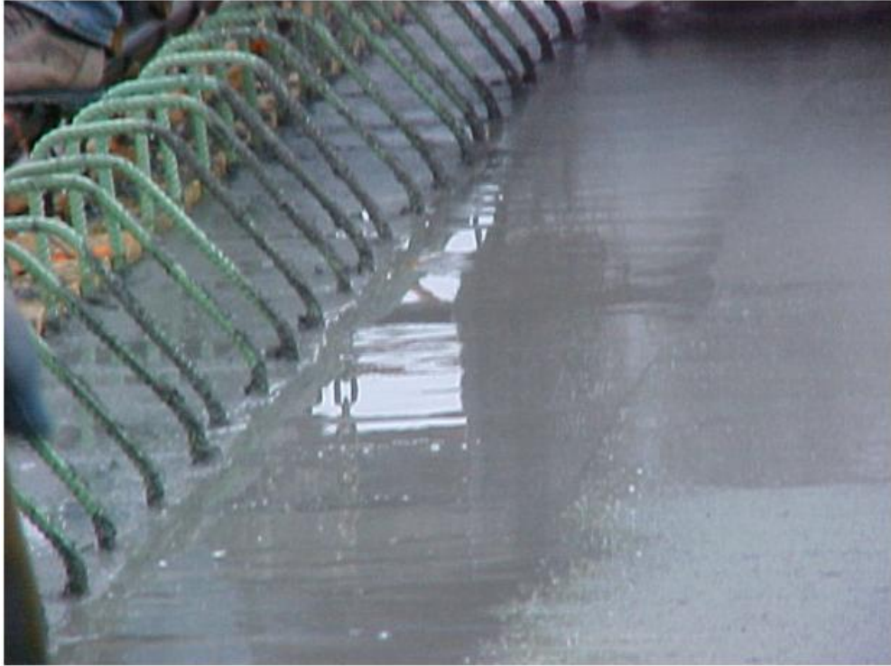
Fig. 8.16 Puddles of Water from Excessive Fogging in Some Patches
