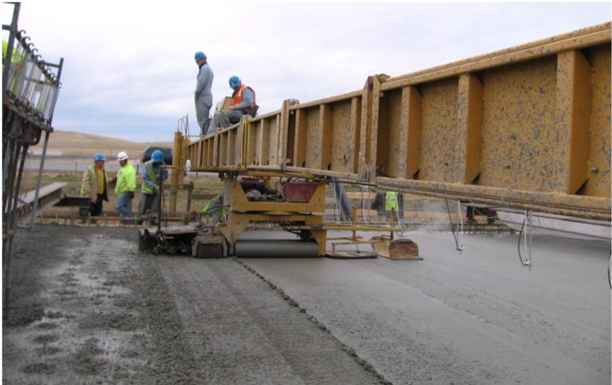
Fig. 8.13 Concrete Finishing with Two Rollers
