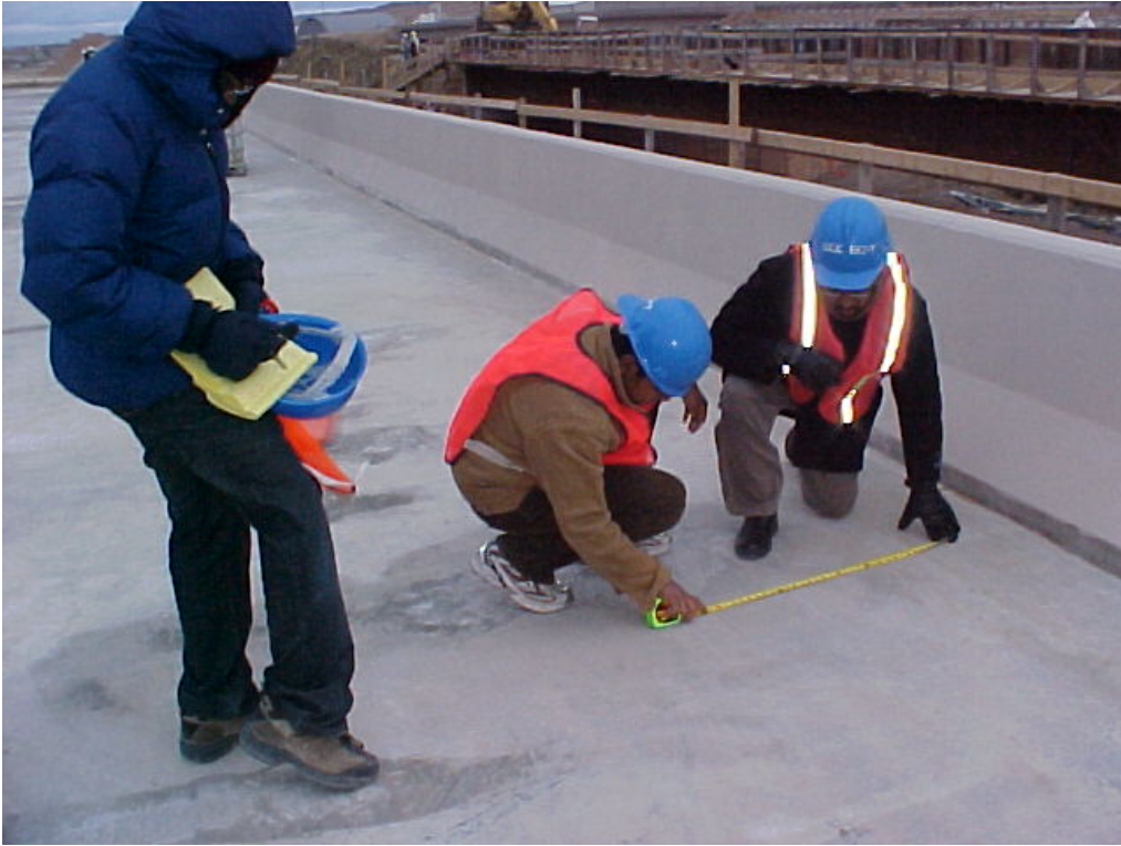
Fig. 9.4 Crack Survey of A45 Concrete Bridge Deck (West Bound)
