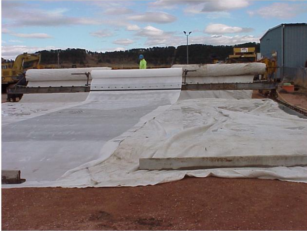
Fig. 8.5 Water Soaked Curing Blankets in Place
