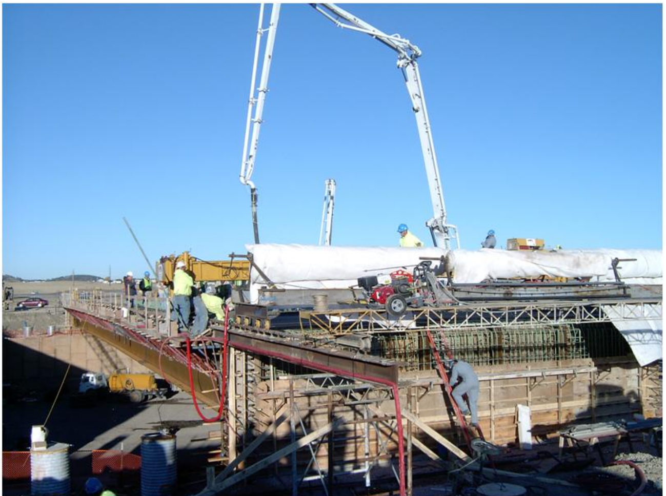
Fig. 8.9 Arrangement for Placing the Curing Blanket in Three Widths
