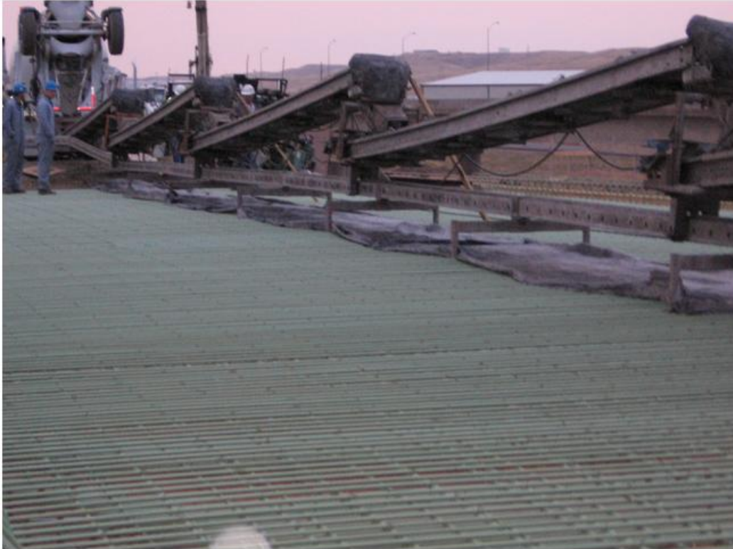
Fig. 8.10 Placement of Concrete with a Conveyor
