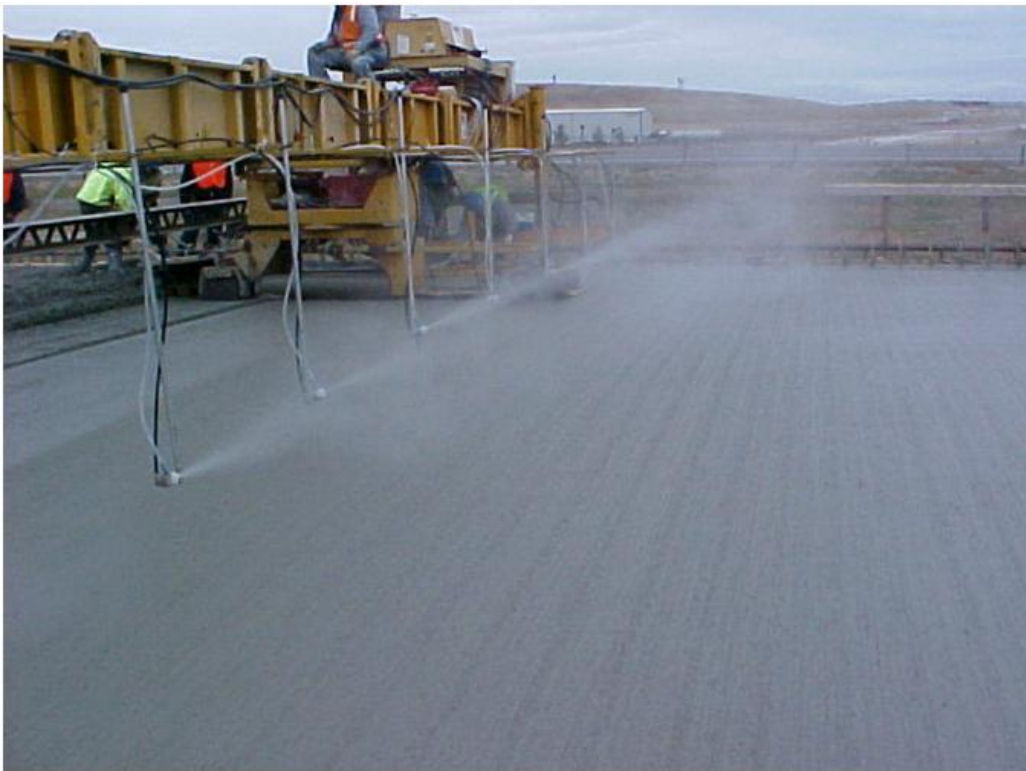
Fig. 8.15 Fogging Arrangement
