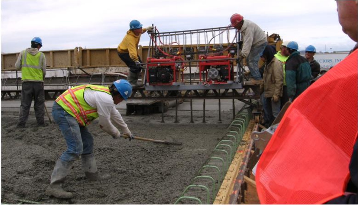
Fig. 8.12 Concrete Consolidation with Vibrators Mounted on a Cross Beam
