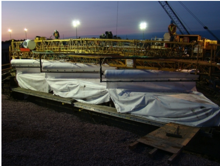
Fig. 8.28 Curing Blankets on the LC-HPC Deck in Brule County
