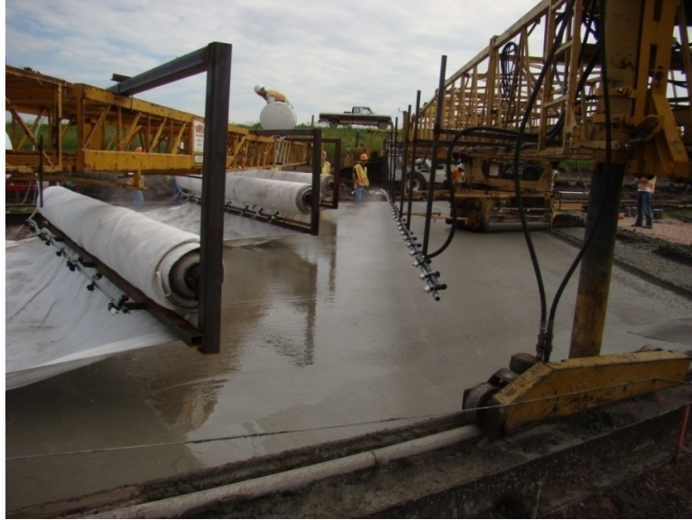
Fig. 8.23 Curing Blankets and Concrete Finish for Test Slab I
