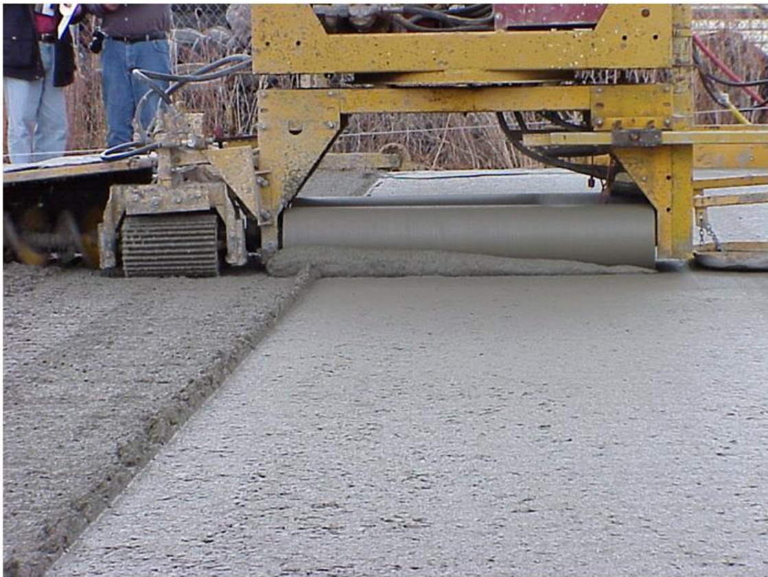
Fig. 8.2 Fines from Concrete Being Excessively Removed by the Roller
