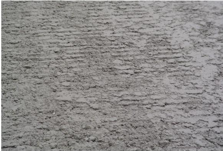
Fig. 8.3 Poor Finish of Concrete
