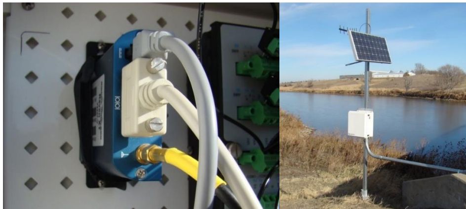
Figure 6-6: Wireless Transmission Modem and Solar Panel Remote Power
