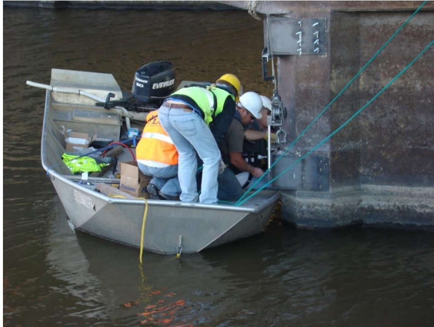
Figure 7-13: Installation of the Monitoring System Cuffs and Anchors
