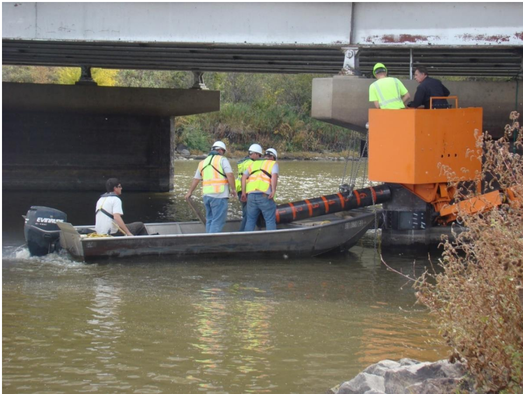
Figure 7-14: Installation of Transducer Pipe at the James River Site
