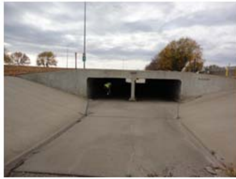
Twin Barrel Box Culvert
