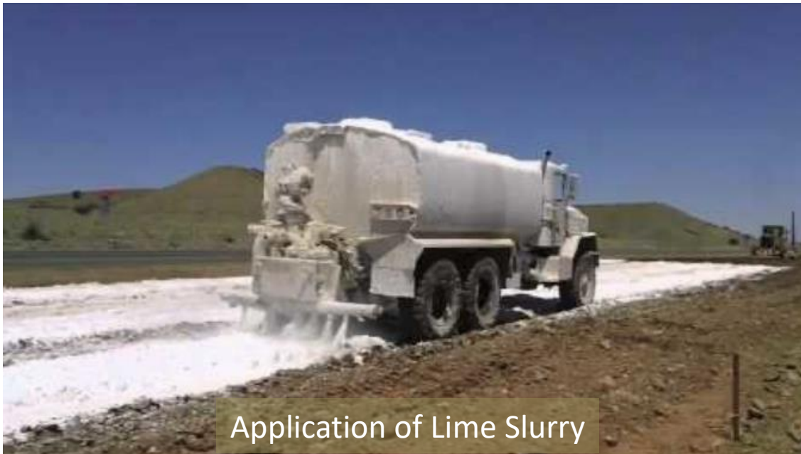
Figure 6 Spreading of Chemical Stabilizing Agent (Portland Cement and Lime) on the Recycled Base Layer for Blending [3]
