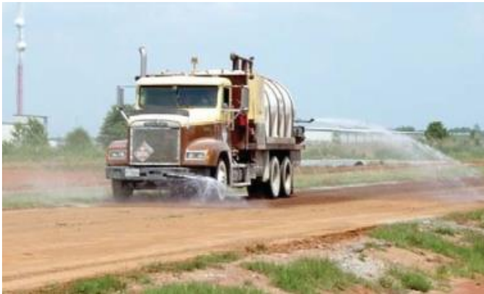
Figure 8 Curing of FDR by Spraying Water [3]
