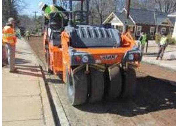
Figure 7 Compaction of the FDR with Tamping Roller, Smooth-Wheeled Vibrating Roller and Pneumatic Tire Roller [3]
