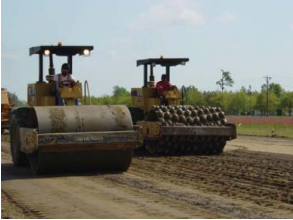
Figure 7 Compaction of the FDR with Tamping Roller, Smooth-Wheeled Vibrating Roller and Pneumatic Tire Roller [3]
