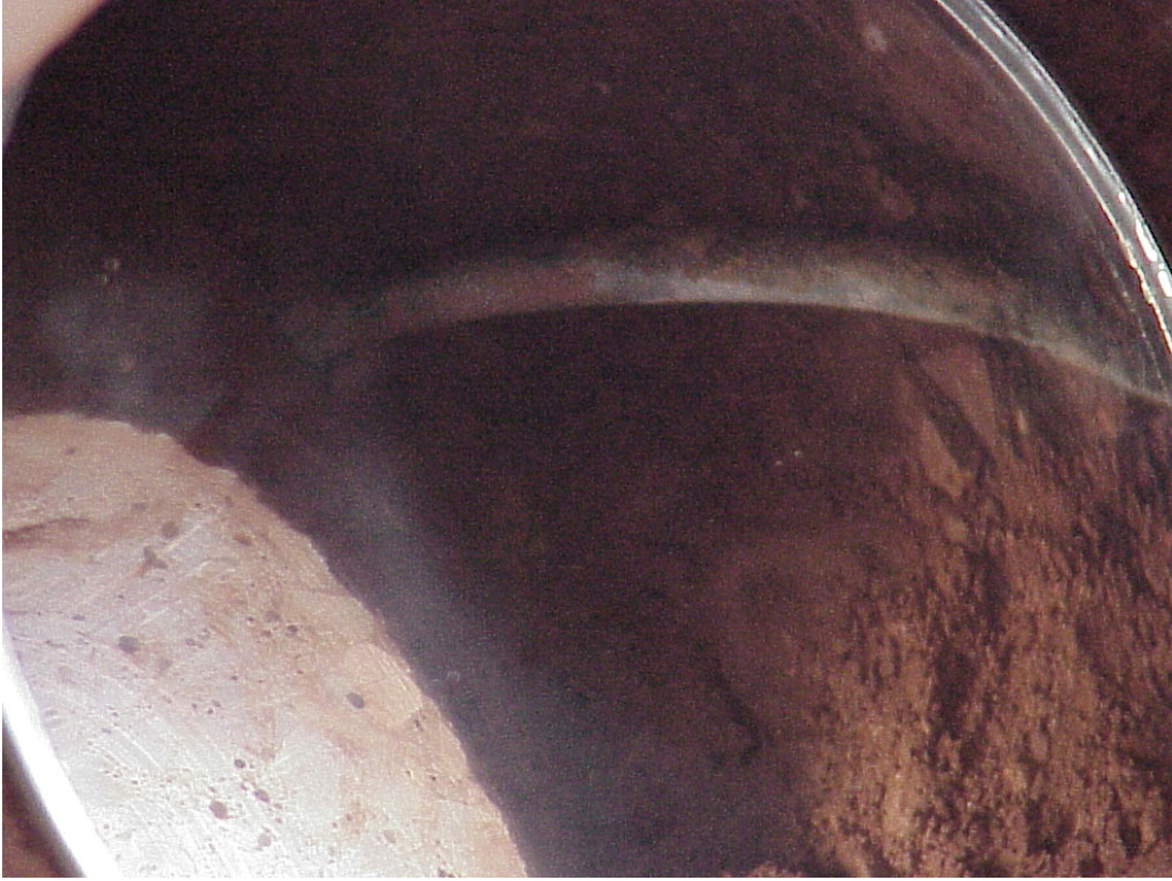
Figure 14 Beginning of bend in mesh at interior wall face station 23+87 left
