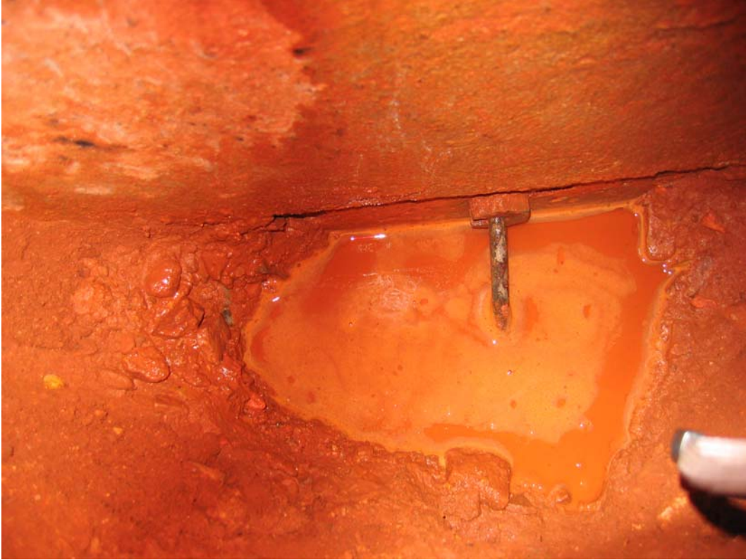
Figure 3 Mesh connector at east abutment of bridge
