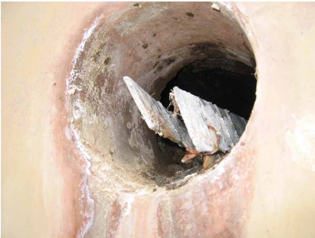
Figure 6 Galvanized reinforcement straps showing zinc reaction product
