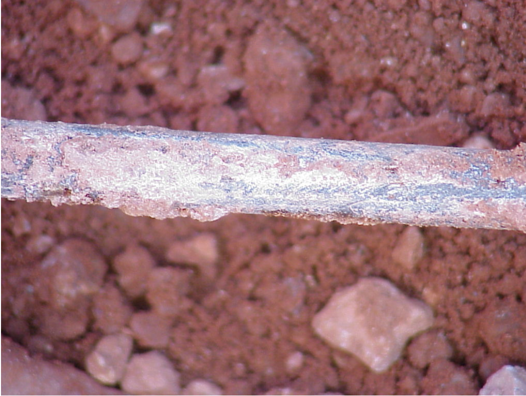
Figure 10 Closeup of reinforcement mesh showing coating of shale/galvanizing
