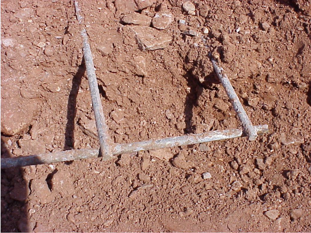
Figure 8 Reinforcement mesh at station 25+89 WB lane
