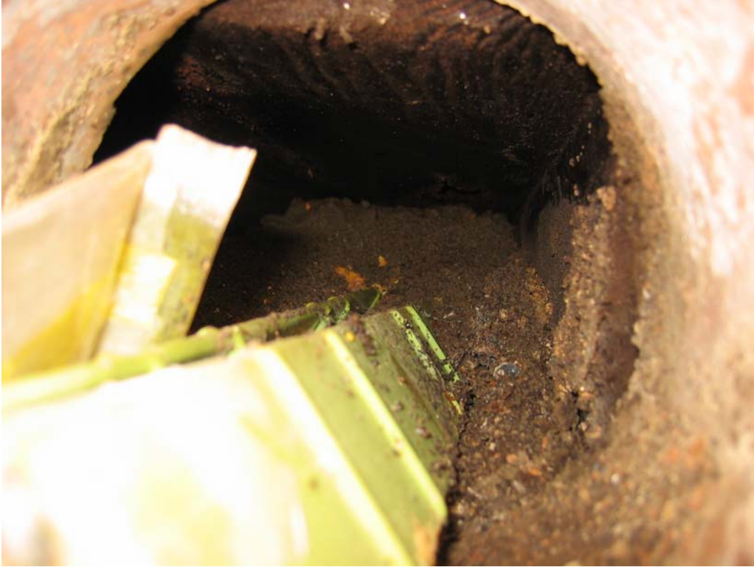
Figure 7 Epoxy-coated reinforcement straps at Deadwood wall
