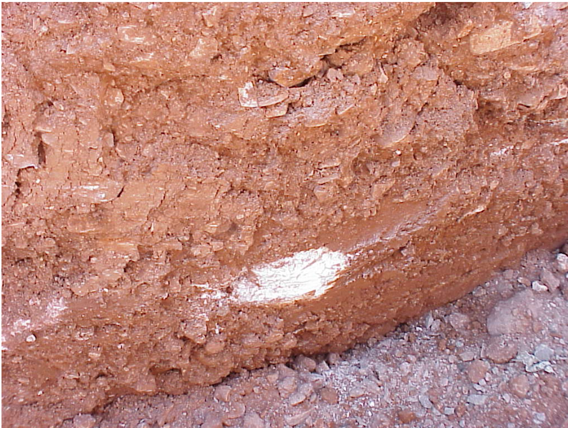
Figure 1 Excavated granular backfill at station 25+44, WBL. Note large gypsum lens.
