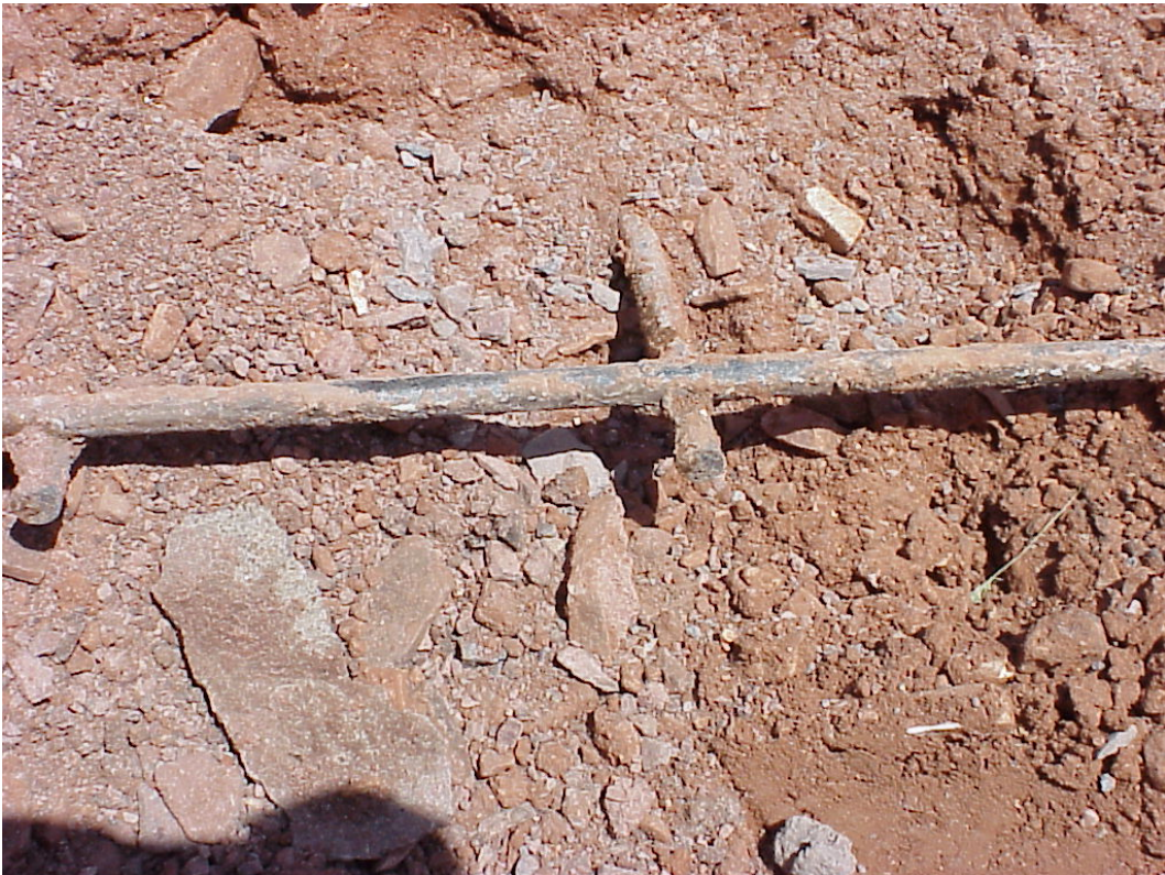
Figure 9 Reinforcement mesh at station 25+44 WB lane
