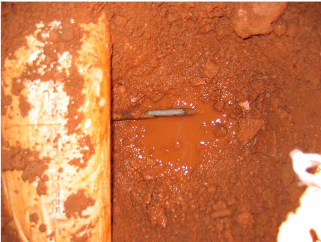
Figure 4 Mesh at southwest corner of west abutment
