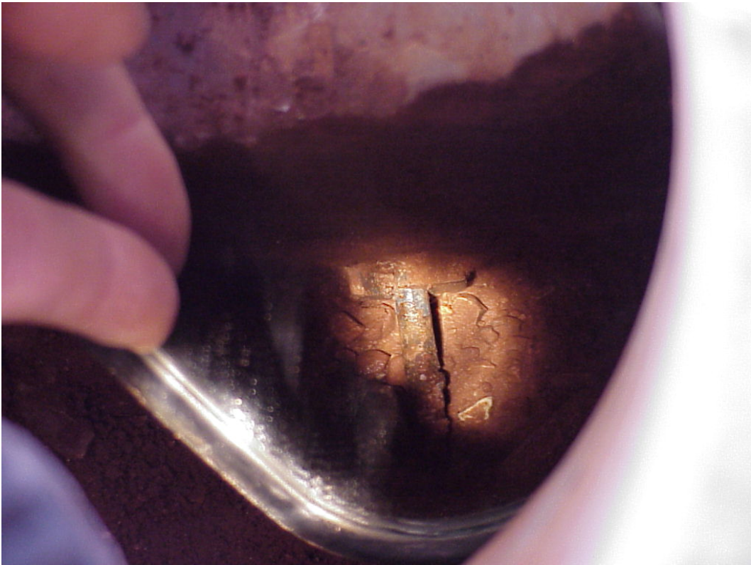
Figure 15 Panel connector near base of wall station 25+89 right
