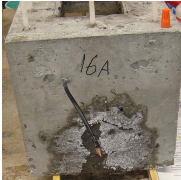
Figure 7-23: Salt crystals from the chloride solution migrating through the concrete.
