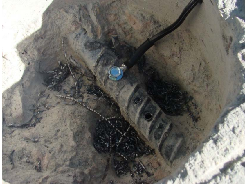
Figure 5-7: Electrical connection to the reinforcing bar
