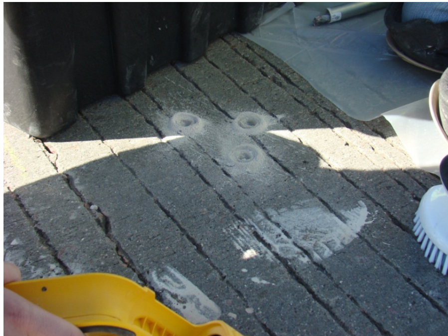
Figure 5-5: Dust created during drilling process
