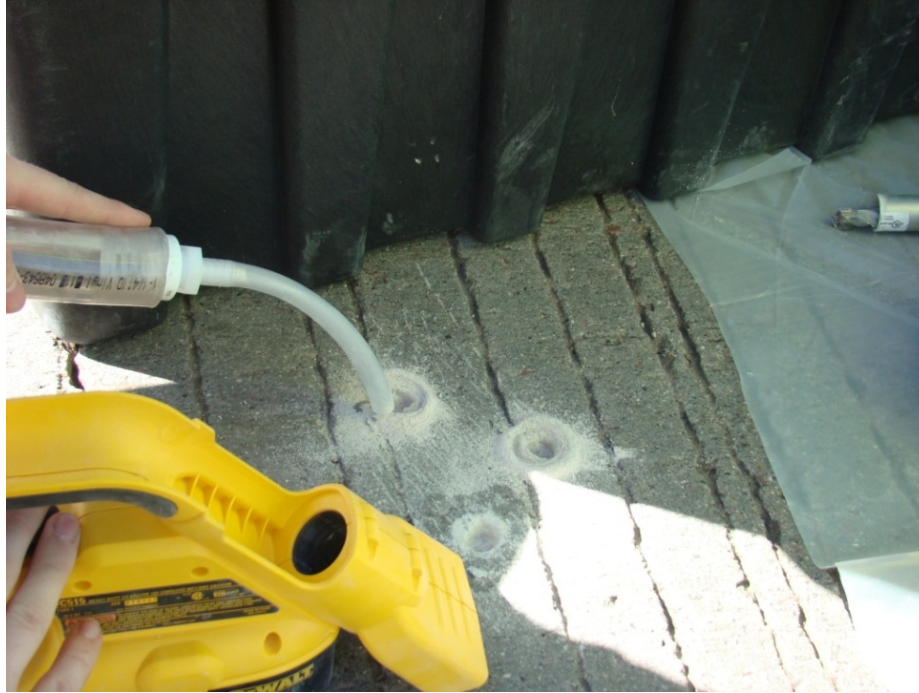
Figure 5-6: Collecting dust from drilled holes
