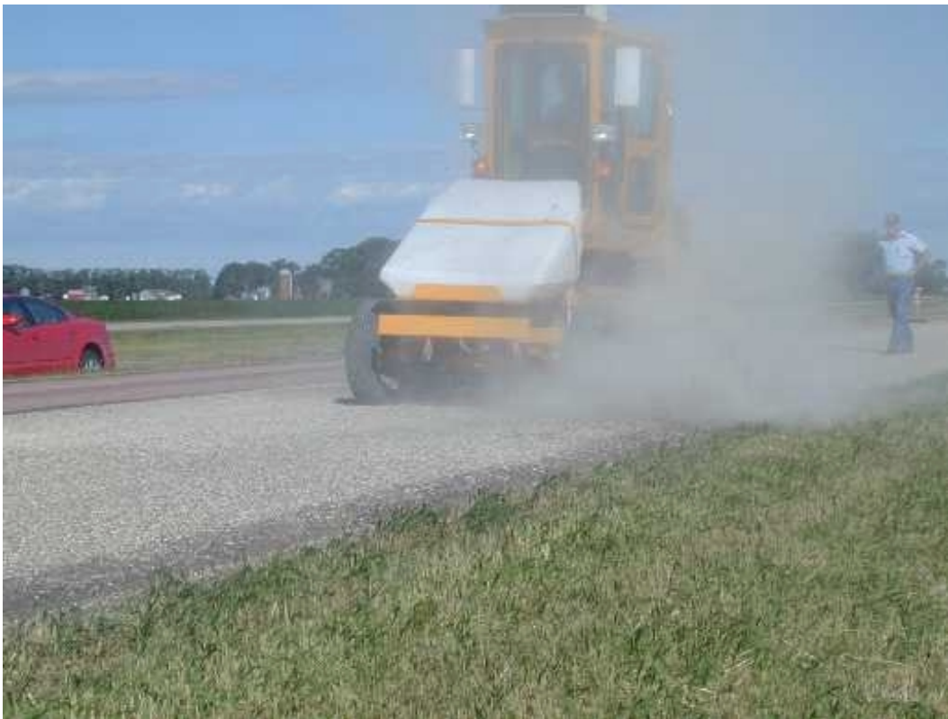
Figure A-16. Sweeping operation (natural aggregate chips).
