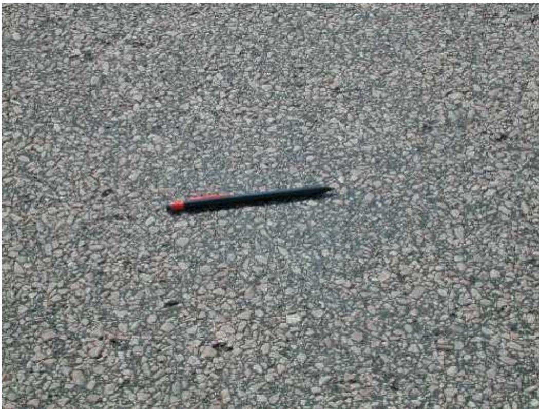
Figure A-2. Typical wheelpath surface texture before chip seal placement.
