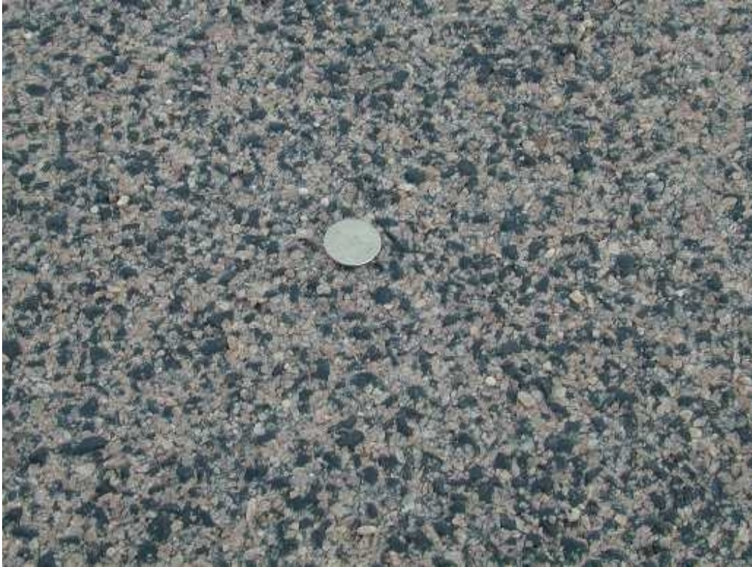
Figure A-13. Choke stone surface (quartzite chips) after opening to traffic.
