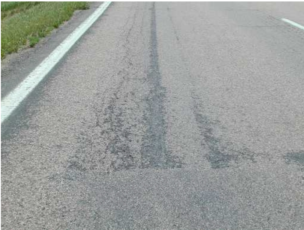
Figure A-4. Medium-severity raveling before chip seal placement.
