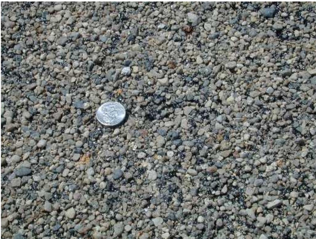
Figure A-14. Choke stone surface (natural aggregate chips) after rolling.
