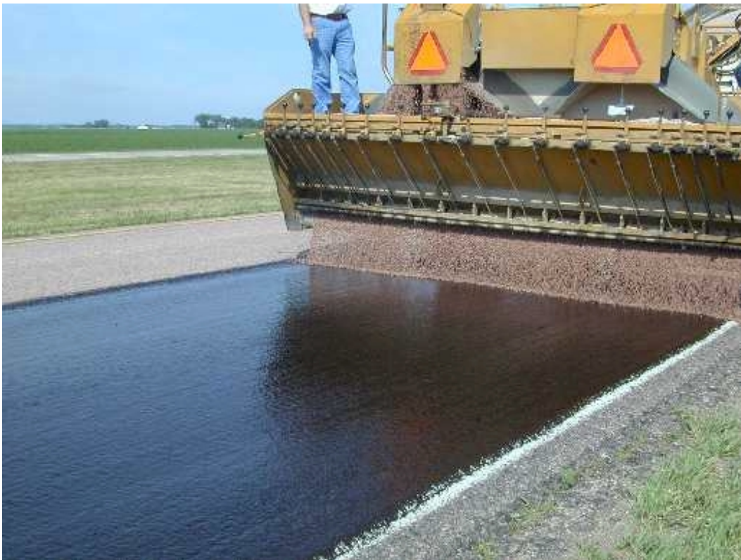
Figure A-10. Application of quartzite chips.
