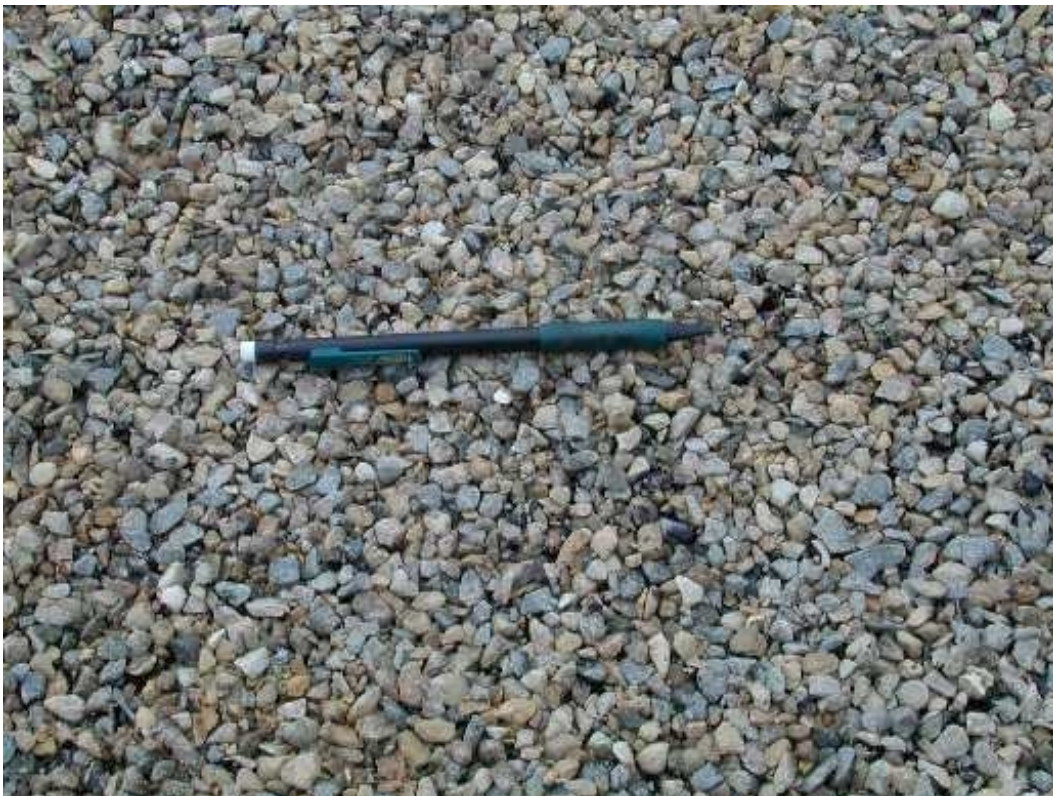
Figure A-12. Close-up of chip seal surface (natural aggregate chips).
