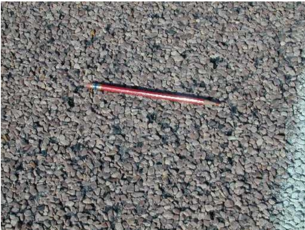
Figure A-24. Missing chips on new design section with quartzite aggregate.
