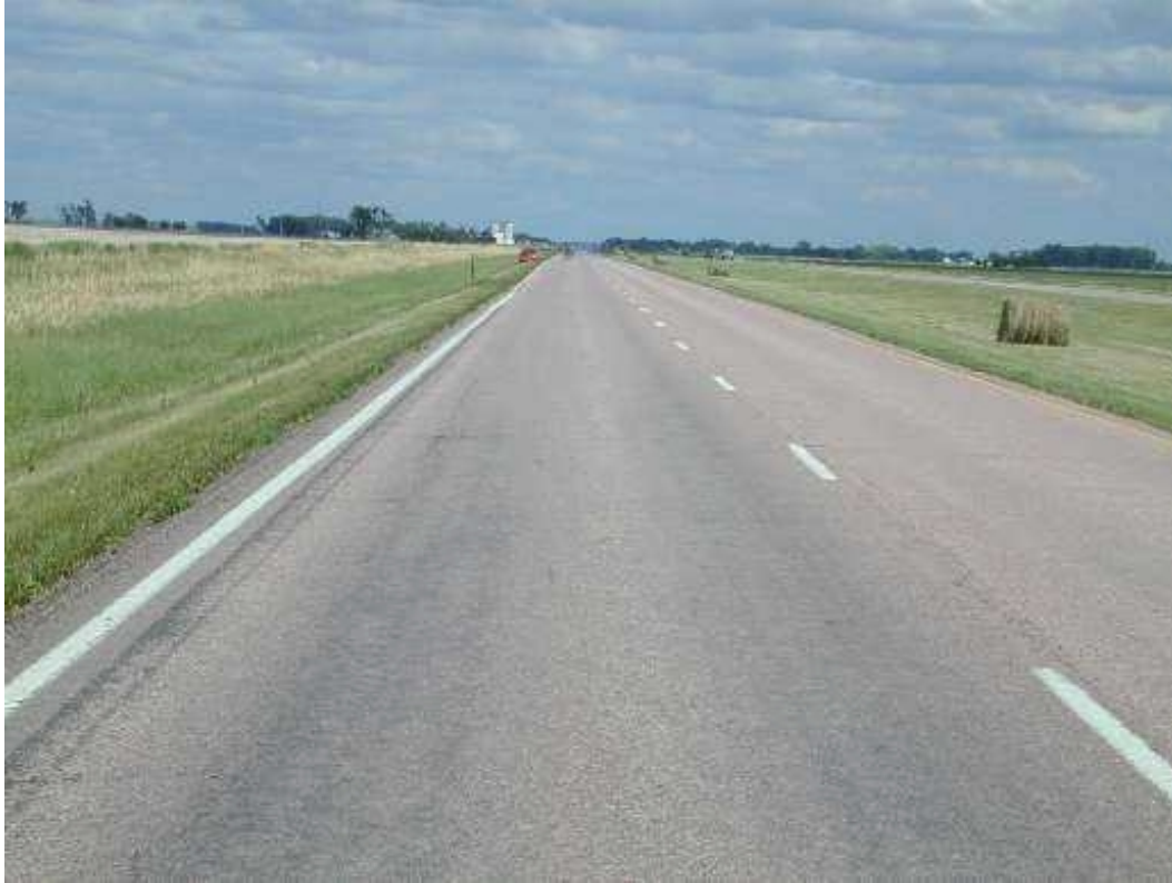
Figure A-1. Typical pavement condition before chip seal placement.
