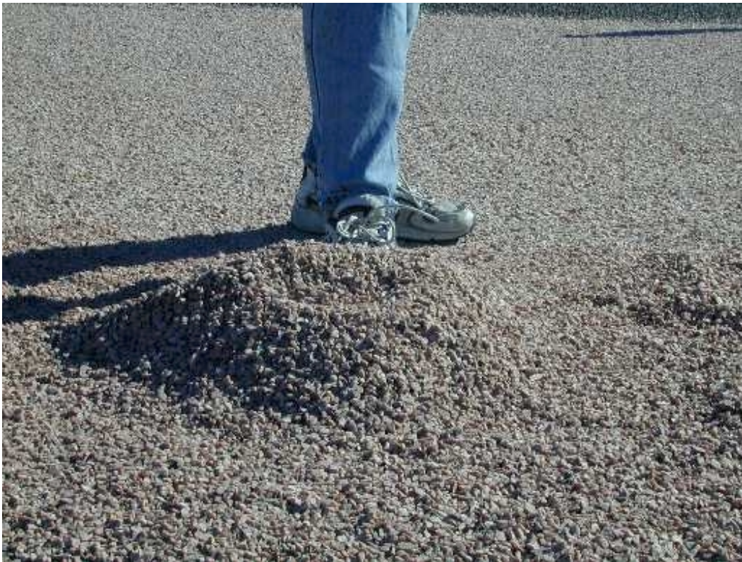
Excess chips after two broom passes (SDDOT standard design).
