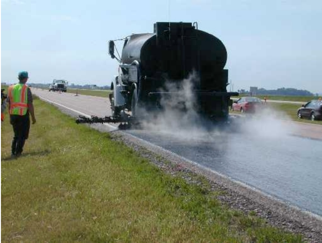
Figure A-9. Application of CRS-2 emulsion.
