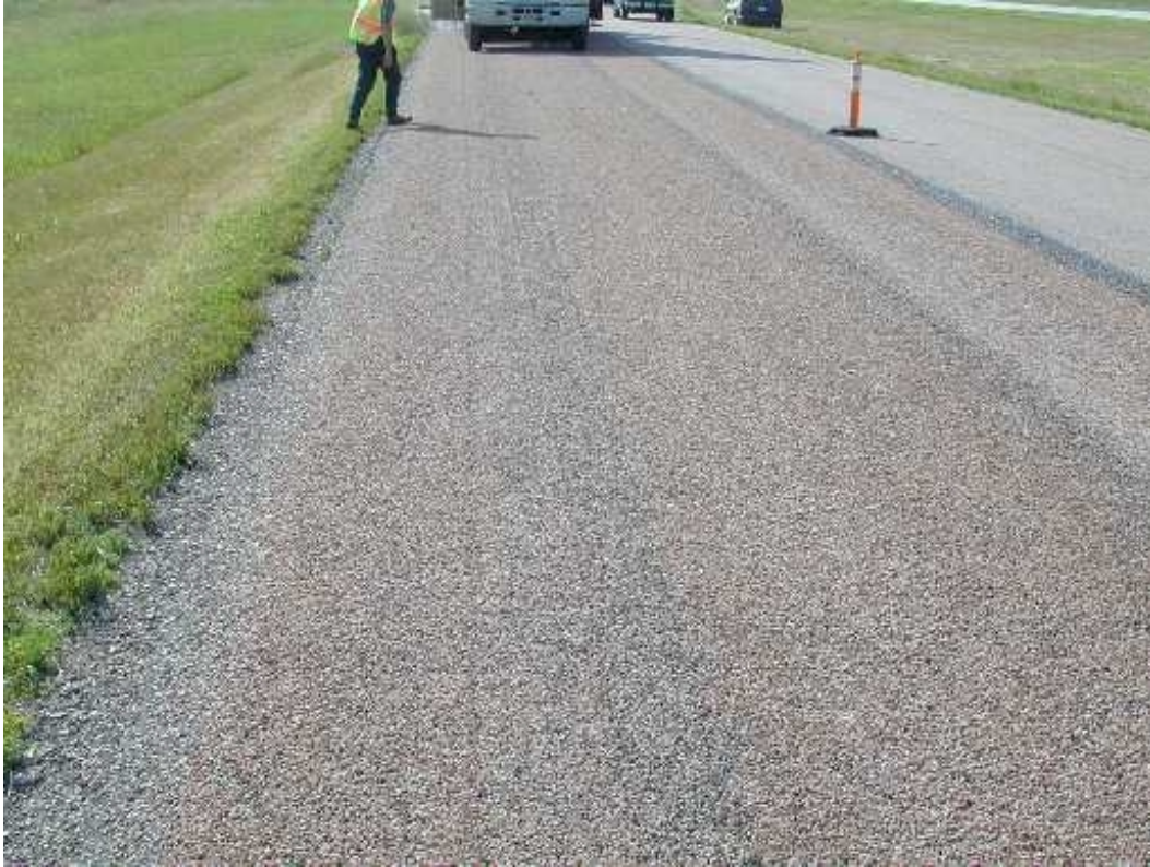
Figure A-11. Chip seal surface (quartzite chips) before rolling.
