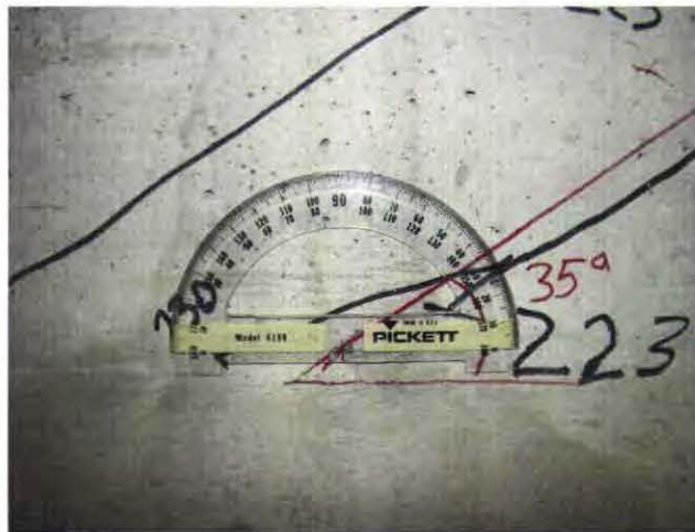
Figure 7.90: Inclination Angle of a Shear Crack
