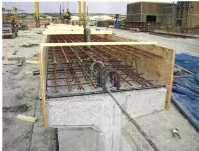
Figure 7.15: Deck Formwork and Reinforcement
