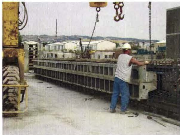
(e) Installation of Formwork
