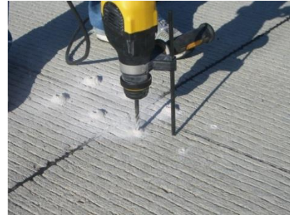
(b) Drilling 5/16" diameter holes
