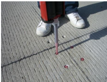
(e) Filling holes with epoxy adhesive
