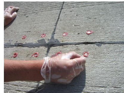
(f) Setting stainless steel bolts inside holes
