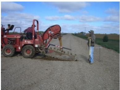
(a) Trenching the subbase
