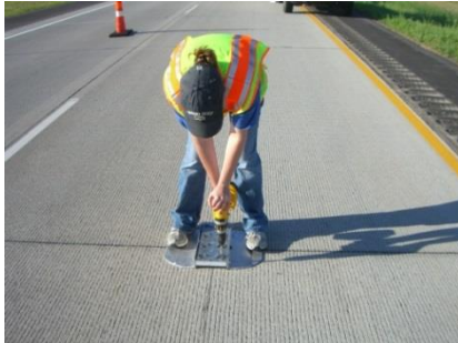
(a) Drilling pilot holes
