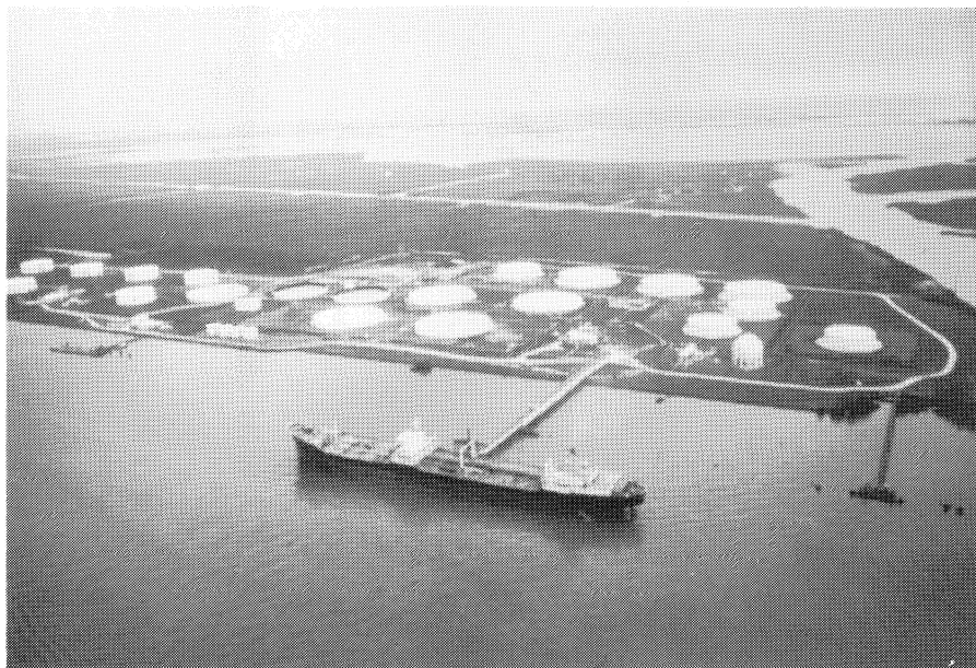
Tanker discharges cargo at Louisiana receiving terminal, providing temporary storage of crude oil for Government's Strategic Petroleum Reserve (SPR). Oil is piped inland to salt caverns for strategic storage. Federal Cargo Preference Act requires that at least 50 percent of SPR oil be carried in U.S.-flag vessels.
