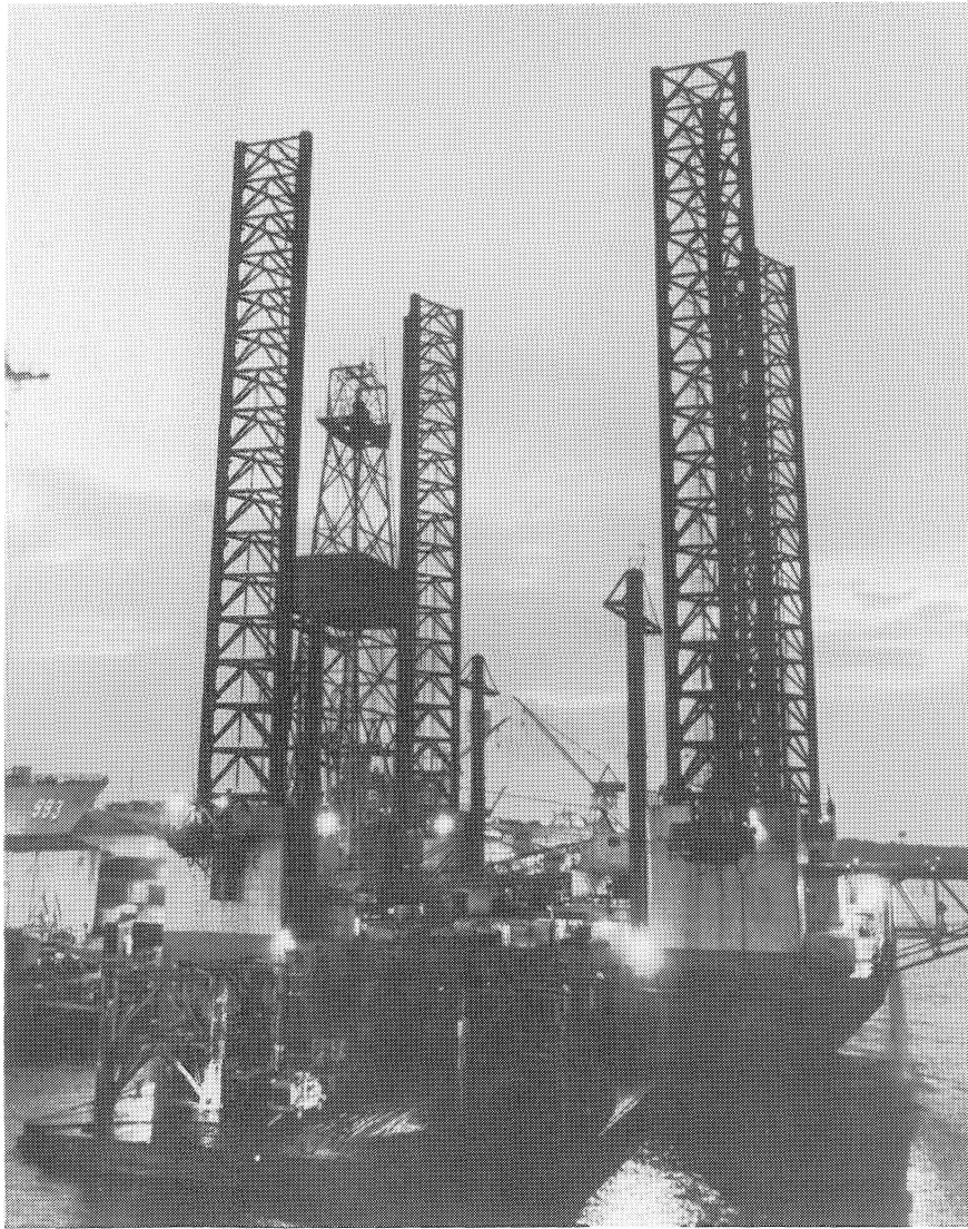
GULFTIDE oil-drilling rig at Pascagoula, Miss., for modification and repair represents re-entry by Litton Industries' Ingalls Shipbuilding Division into offshore activities.
