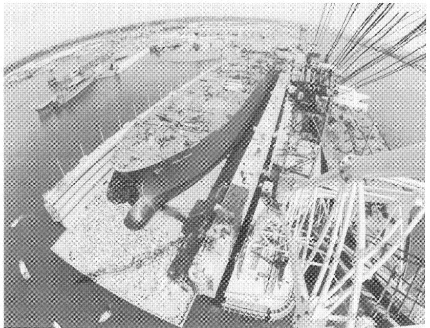
Fisheye lens view of MOBIL ARCTIC under repair in Portland's Dry Dock 4, at 982 feet largest floating dry dock on West Coast. Photo was made at "People's Day" open house May 19, 1979.
