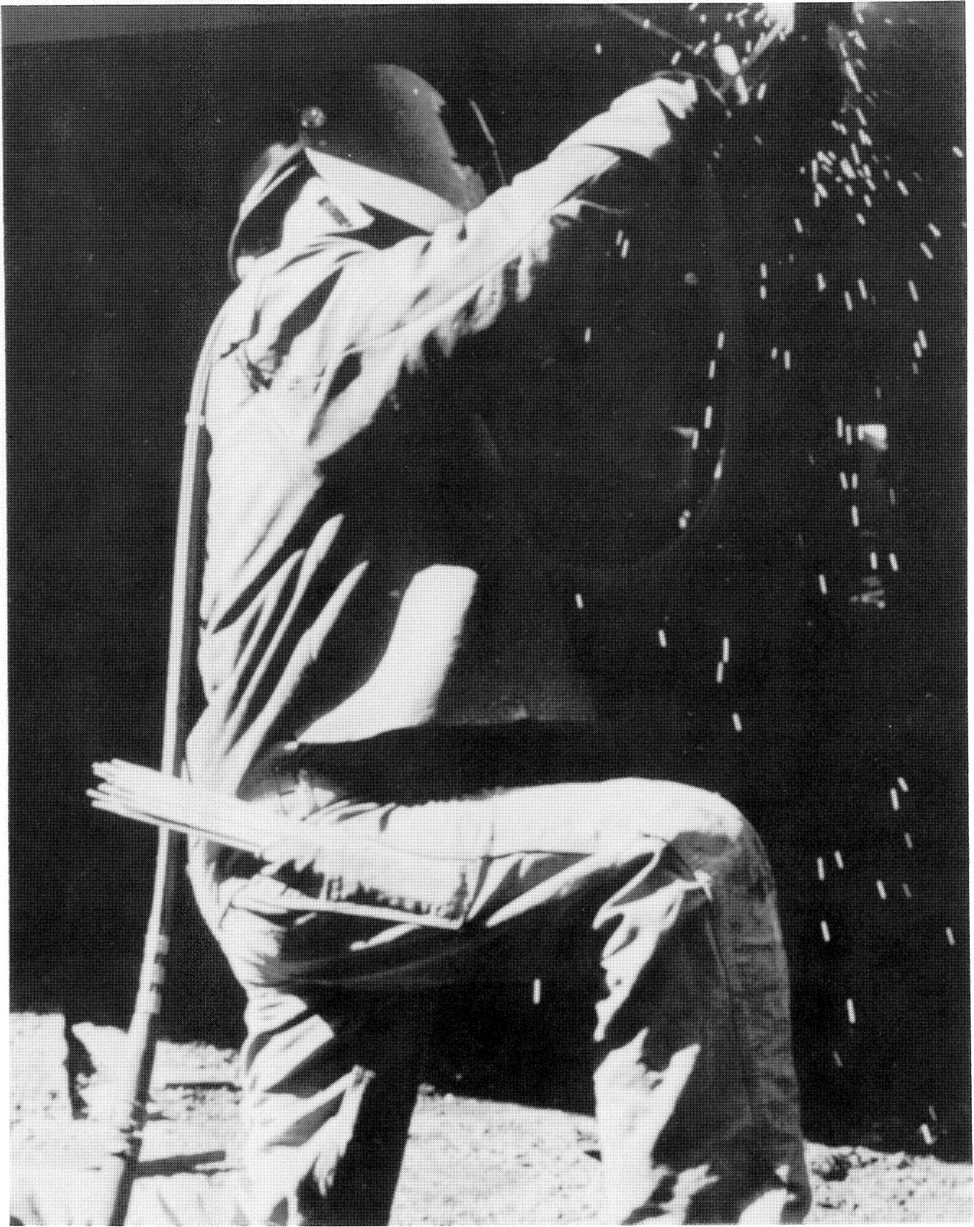
Welder at work on bottom plates of ship's hull in drydock at Todd Shipbuilding's Seattle (Wash.) Division.
