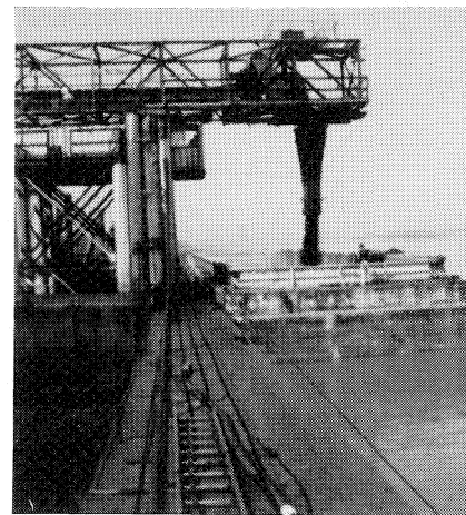
Coal moves from railroad car (not shown) on conveyor belt (top) into barge at American Terminal operated by American Commercial Barge Line Co. on the Ohio River at Louisville, Ky. Coal transfer system is one of four operated by company on Ohio and Mississippi Rivers.
