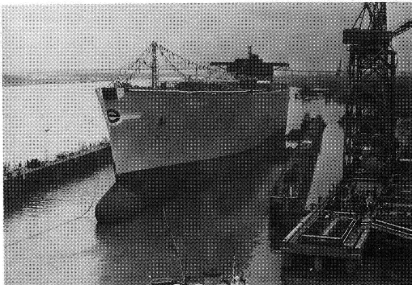
Hull of EL PASO COLUMBIA, one of 18 liquefied natural gas carriers under construction in U.S., is launched from Avondale Shipyards, Inc., New Orleans, La. Hull was then taken to outfitting berth to be prepared for delivery to owner.
