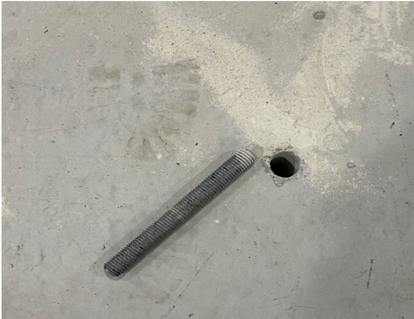
Figure 2.5 Nonproprietary shear anchor prior to installation
