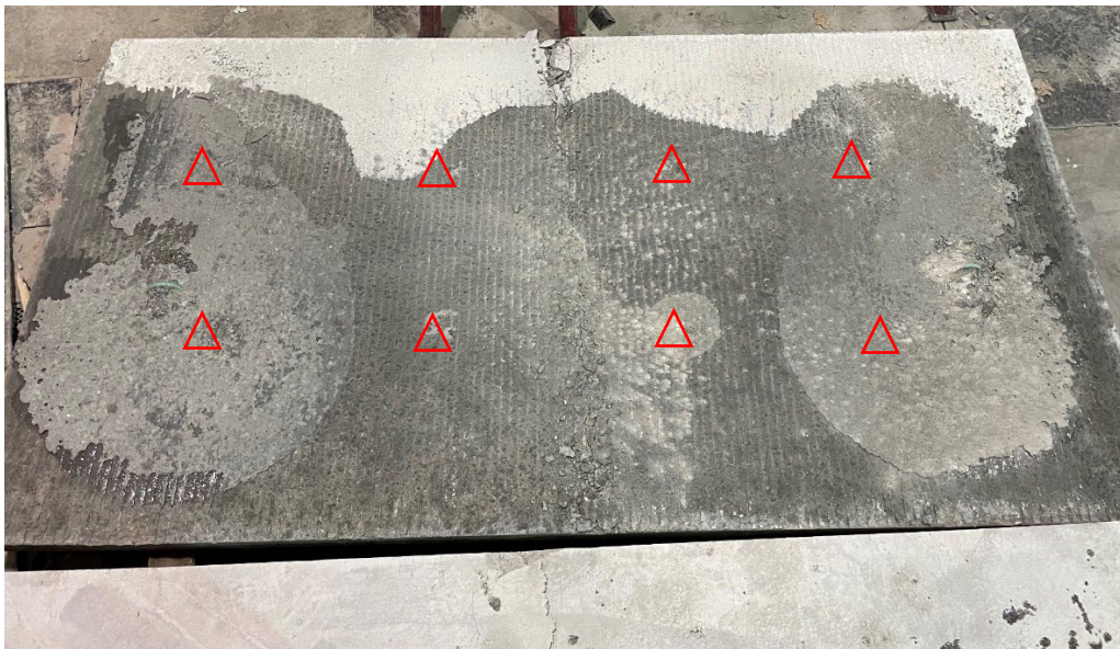
Figure 3.10 Distribution of epoxy after testing on the precast panel surface (Triangles indicate location of the epoxy injection sites)
