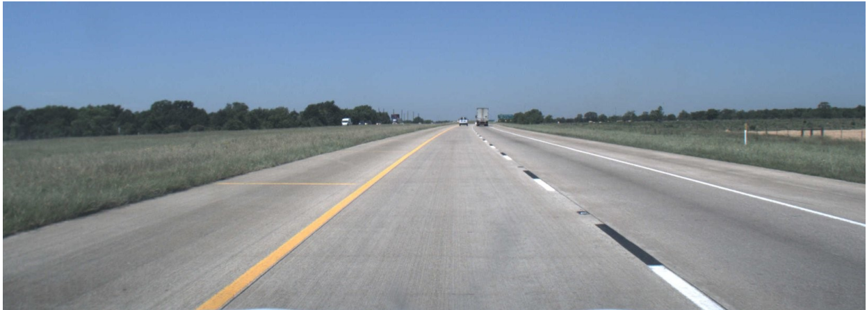
Figure 4. Image of a road segment with white pavement marking followed by black (driving westbound).
