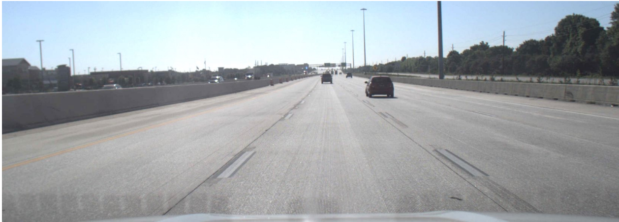
Figure 7. Image of a road segment with white pavement markings with a black border (driving eastbound).
