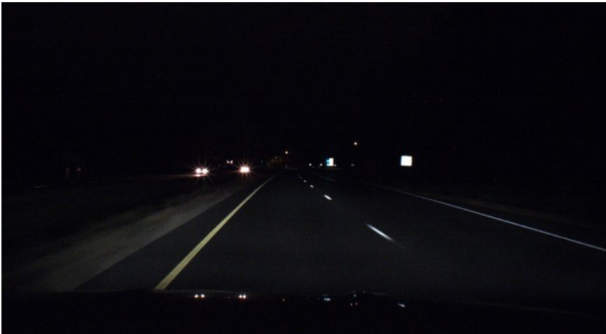
Figure 47. Test site 5a.
