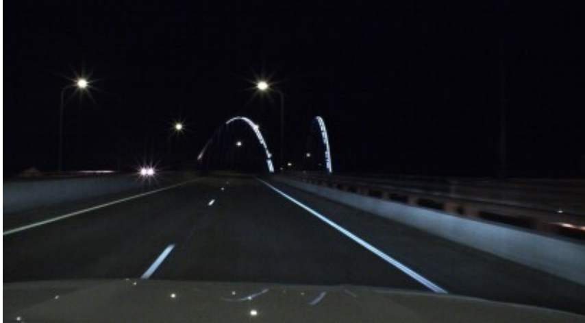
Figure 67. Test site 32a.
