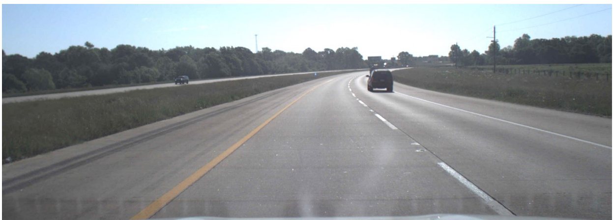
Figure 5. Image of a road segment with white pavement marking followed by black (driving eastbound).
